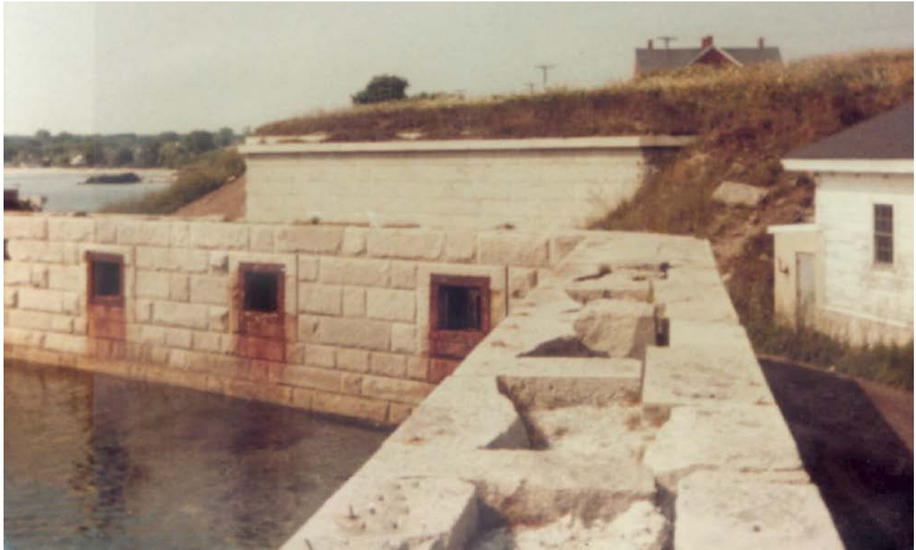
Unfinished scarp of the new Fort Preble. A portion of the old fort's scarp is visible in the background. Author
