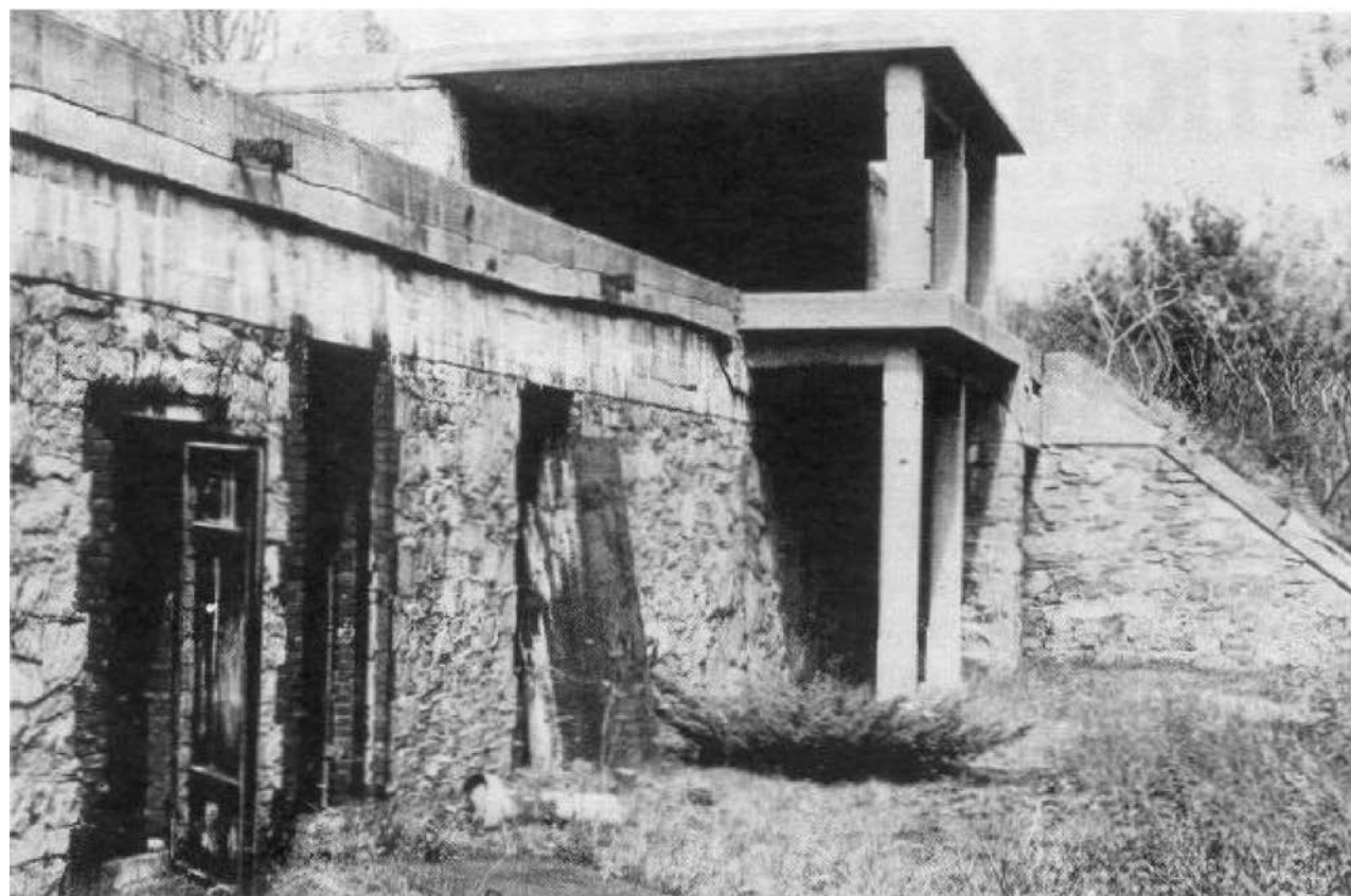
Portions of Battery Thompson were constructed with a facade of native stone. Author's Collection
