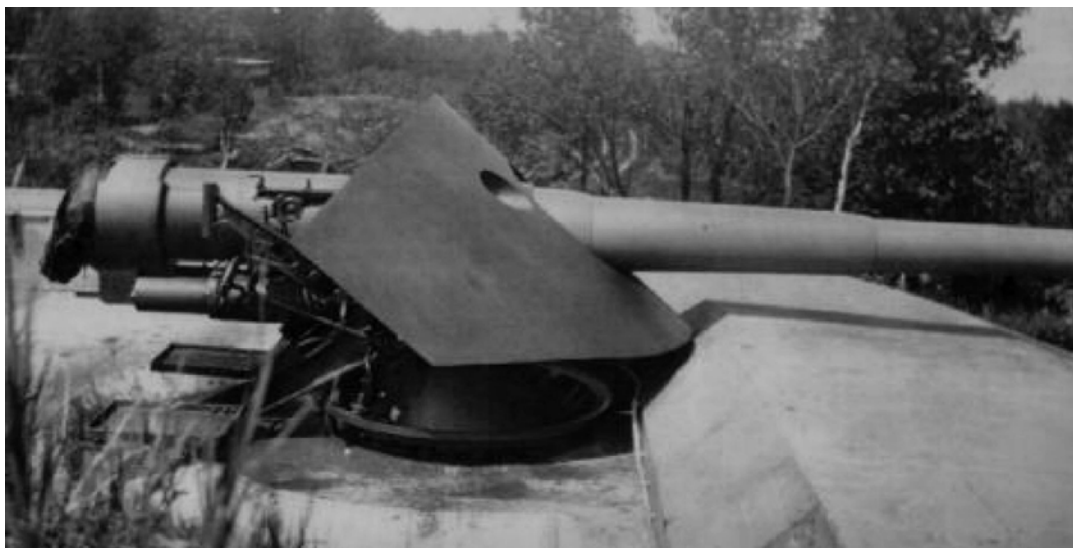
M1900 6-inch R-F gun mounted on M1900 barbette carriage. Author's Collection
