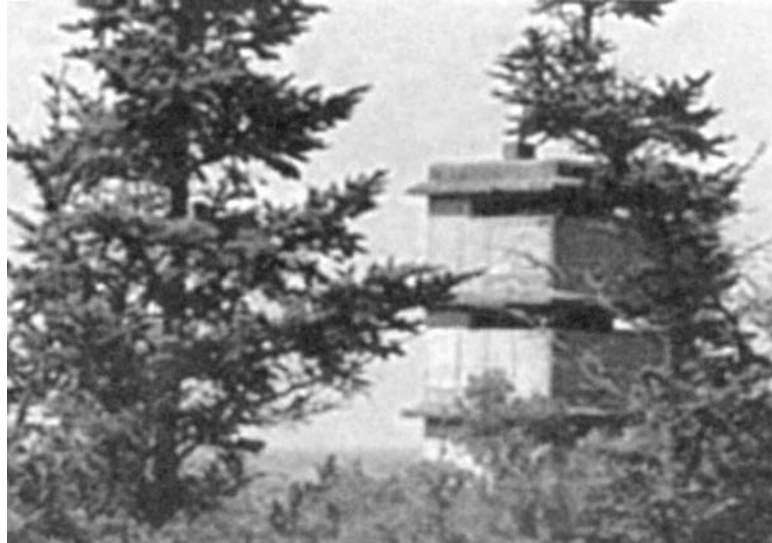
The three observation levels of Jewell Island's 8-story base end station. Author's collection
