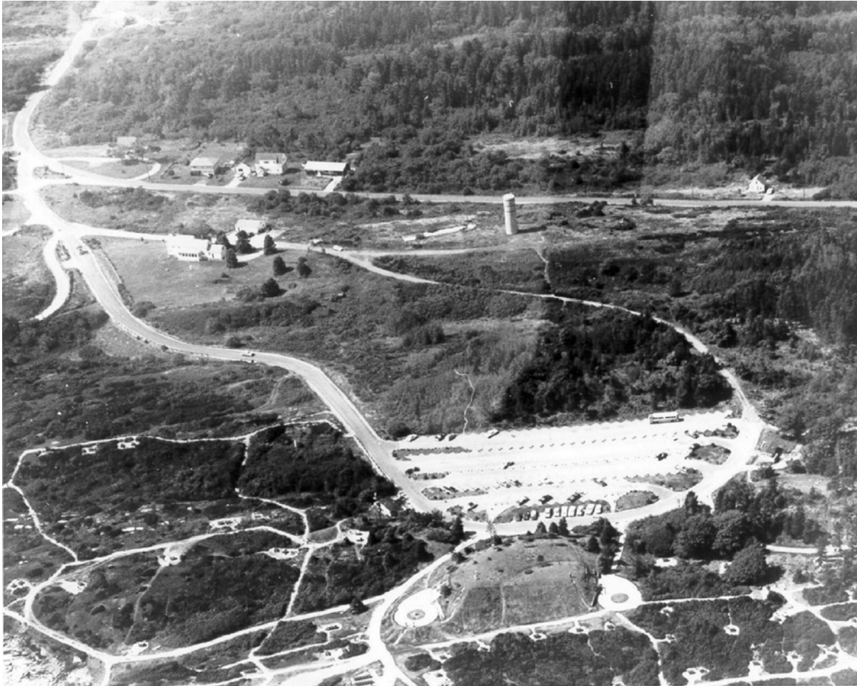
Cape Elizabeth State Park, ca. 1960. BCN 201 is in foreground and the six-story fire control tower in upper center. Courtesy of E.R. Lewis
