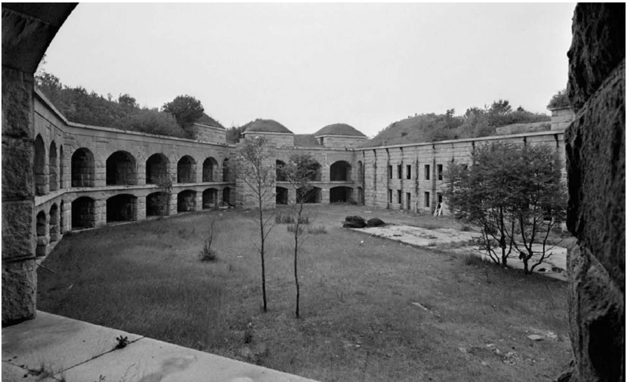
Parade of Fort Gorges 1930. Note the bombproof magazines on the barbette tier. Gorge is at right. HABS
