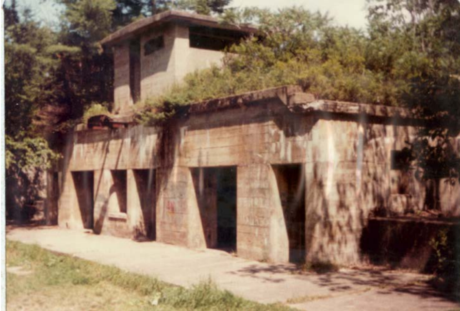
The central traverse of Battery Cogan, surmounted by the combination BCS and CRF station. Author
