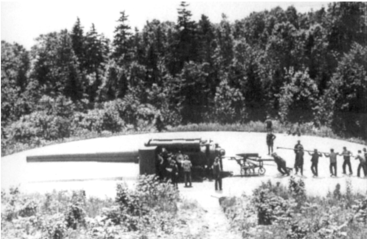
Battery Foote's Gun No. 1 at loading practice. Private collection
