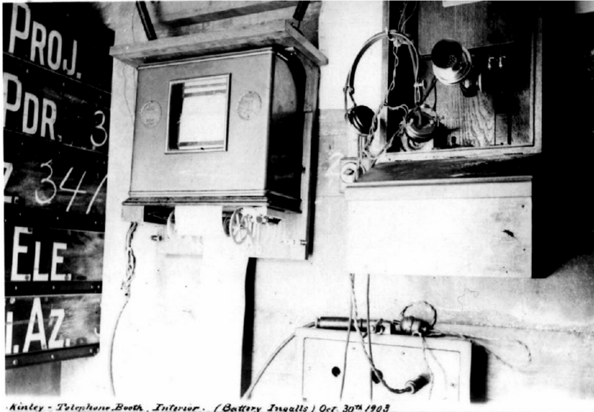
Interior of Battery Ingalls' telephone booth. Note the firing data board at left. NARA
