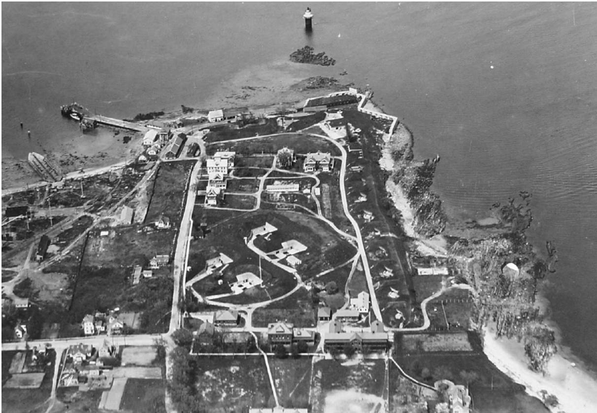
Battery Kearny's four pits occupied much of the central portion of Fort Preble. NARA
