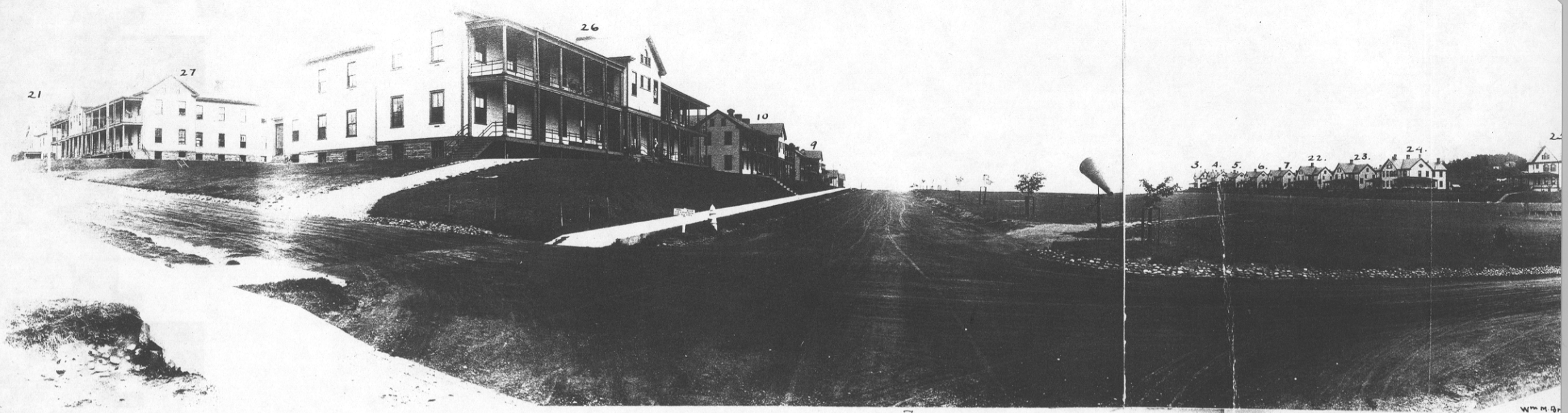
BARRACKS 21-27-26-10-9. OFF. QRS. 3-4-5-6- 7 22-23-24-25. LOOKING EAST FROM GUARDHOUSE.
