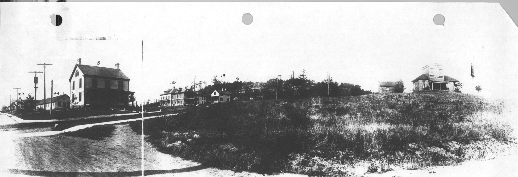
W m M. Britton BARRACK 27.- ART'Y ENG'R STOREHOUSE 44.- OLD HEADQ'RS 8.- HOSPITAL 18.- HOSP. STEWARD'S Q'RS 19. FORMER RESIDENCE OF BRITISH CONSUL ALEXANDER ON RIGHT. HAS WATER TANK IN TOWER. TAKEN SEPT. 1913.
