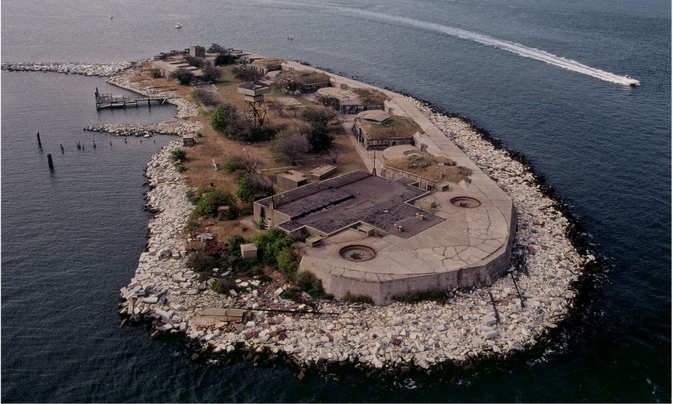
Historic Fort Wool before conversion to seabird nesting habitats
