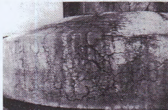
Fig. A.1.6f-Pattern cracking (alkali-carbonate reaction)
