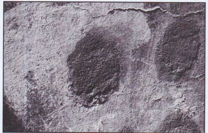
Removing core leaves a large hole that must be repaired. This repair needs to be resurfaced so that it will better match the surrounding historic fabric. Battery Worth.
