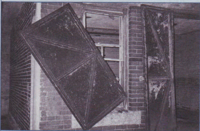
Figure 2. A portion of the 1902 brick mining casemate as it appeared in 1996, with one of the steel window shutters askew. The walls and ceiling of the concrete shell are visible, as is the air space that surrounds the brick walls.
