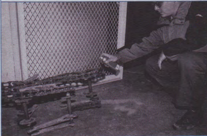
Washington State Parks ranger Evan Roberts applies a corrosion inhibitor to help preserve metal work on an disassembled ammunition hoist at Fort Columbia State Park.
