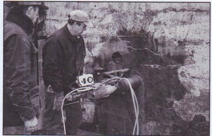
Both water and power are required to operate a coring machine. Battery Worth, Fort Casey, Washington.
