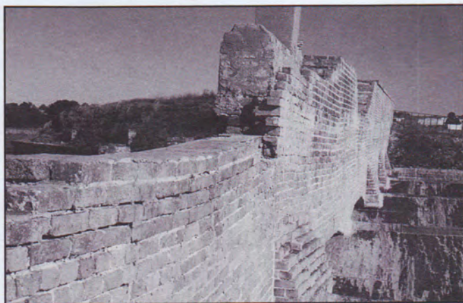
The earth fill behind this masonry wall has been removed. The wall was not designed to stand alone, and it is now unstable and vulnerable to collapse. Fort Pickens, Florida.
