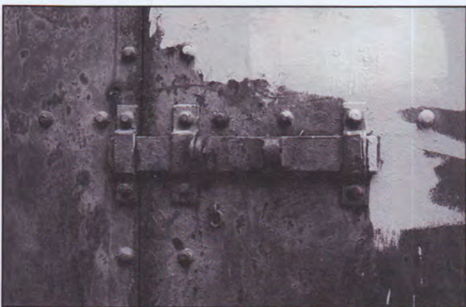
An operating slide secures this double-leaf door. The nut is welded to the bolt that passes through the padlock opening, but no part of the slide itself is welded. Periodic lubrication will ensure its continued functioning.
