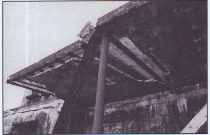
Several causes contributed to the failure of this platform at Battery Cullum at Fort Pickens. Included among them are loss of a supporting column, corrosion-induced loss of section in the beam, and questionable original design detail.
