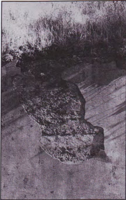
The sub-standard condition of this parge coat could have been detected by simple acoustic impact tests. Battery Cavallo, Fort Baker, California.
