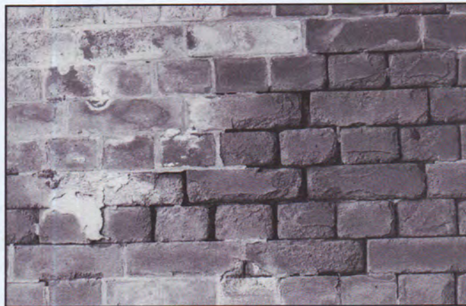
Open joints indicate that this brick wall is overdue for repointing. Battery Cavallo, Fort Baker, California.
