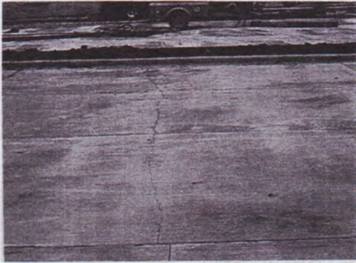
Fig. A.1.8-Shrinkage cracking
