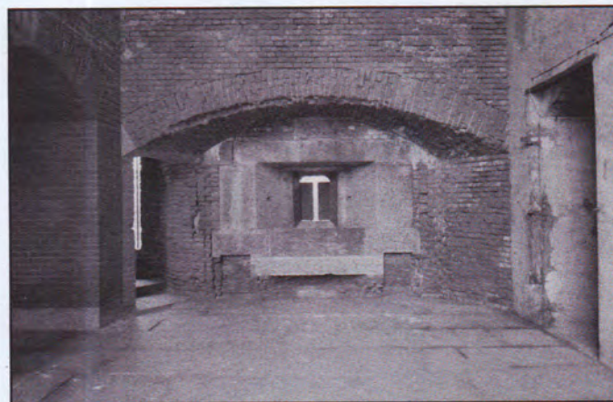
Casemate interior looking toward the embrasure that has been fitted with iron shutters. Fort Delaware, Pea Patch Island, Delaware.
