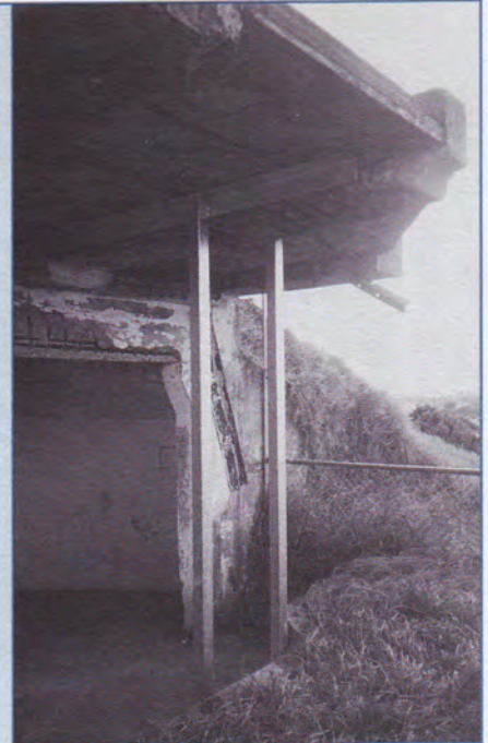
Figure 3. Steel supports for emplacement roof, North Head.
