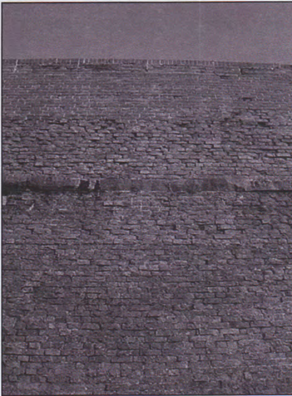
Exterior wall surface in fair to poor condition—note large percentage of open wall joints and eroded surface of bricks.
