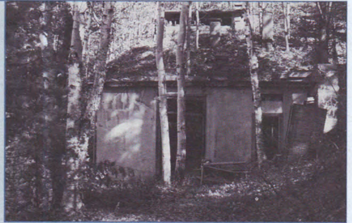
Figure 3. The 1909 wood frame addition to the mining casemate as it appeared in 1996, with the wing on the right collapsed. The earth cover of the 1902 mine casemate is visible above the addition with the 1920 range finder station on top.
