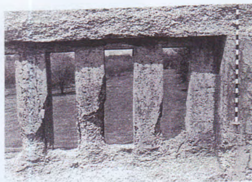
Fig. A.2.20.4a-Scaling (very severe)
