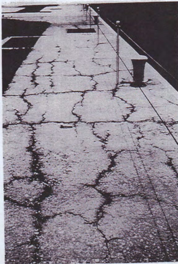
Fig. A.1.6d-Pattern cracking (alkali-silica reaction)
