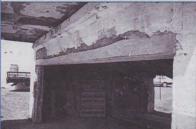
Figure 7. New plaster in place on main lintel, Fort Takapuna.
