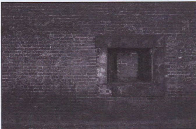
The dark area at the point of ground contact indicates rising damp. As the name suggests, the condition moves moisture upward as a result of capillary attraction. Fort Point, California.
