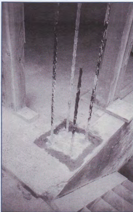
Figure 6. The deteriorated column was removed with careful saw cuts as well as power and hand hammers, leaving as much original rebar as possible.
