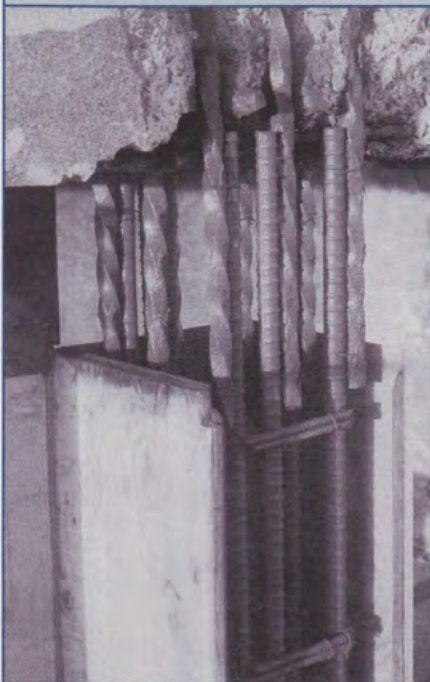
Figure 7. Replacement and original reinforcing rods are coated and tied together prior to pouring rapid setting concrete.
