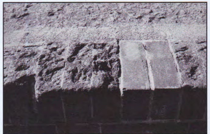
These two new bricks replaced damaged units. Avoid distressing new material to give it the appearance of age. Fort Point, California.
