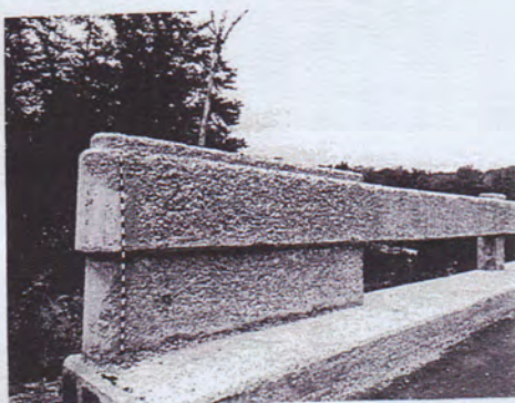
Fig. A.2.20.3a-Scaling (severe)
