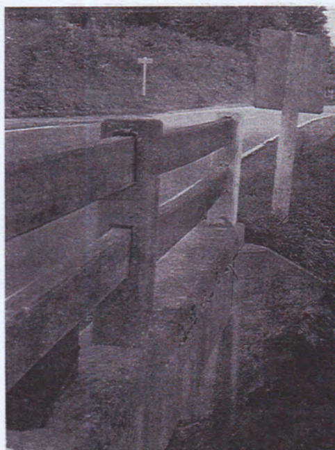
Fig. A.2.10-Distortion
