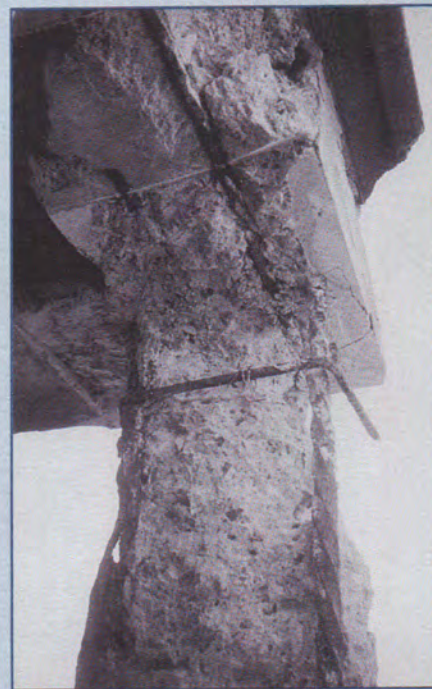
Figure 5. Severe spalling of vertical pillar supporting overhead protection at ammunition hoist, 2000.
