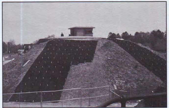
The geotechnical properties of soil were not thoroughly understood when many fortifications were built. An environmental mat helps stabilize the soil on this steep slope. Battery Gregg, Fort Mott, New Jersey.
