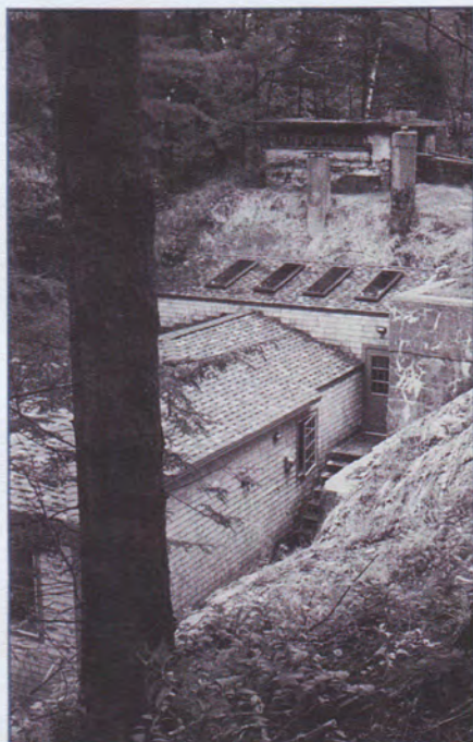
Figure 5. A view of the new residence built on the foot print of the 1909 addition. The connection to the earth-covered 1902 mining casemate is visible, as is the range finder station.
