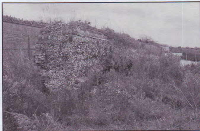
This lightly compacted mixture of a tabby-like material provides in-fill for the masonry walls of Fort Livingston, Louisiana.
