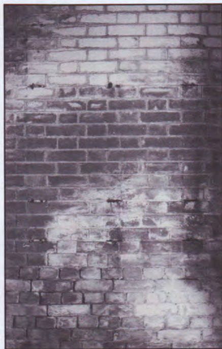
The appearance of crystalized salts is referred to as efflorescence. Battery Cavallo, Fort Baker, California.
