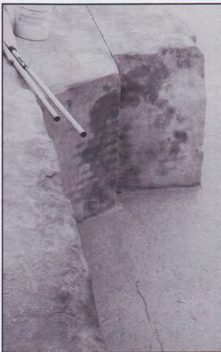
Close-up view of a new stucco application and an elastomeric membrane at Fort Sumter, South Carolina.
