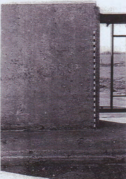
Fig. A.2.20.1a-Scaling (light)
