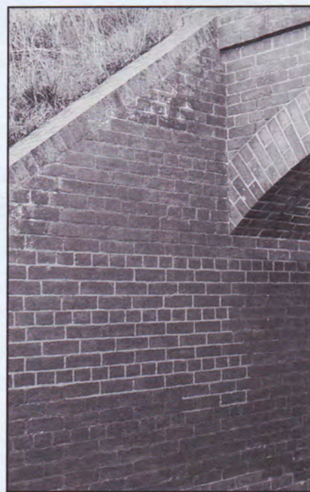
If the repointing mortar does not match the appearance of the existing mortar, the repair will be too noticeable. Battery Cavallo.
