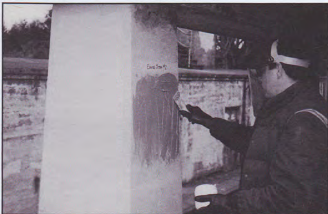
Ranger Todd Jensen experiments with a commercial graffiti remover during cold-weather tests at Fort Worden, Washington. These preparations are often caustic, and protective clothing should be worn.
