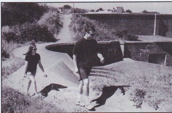
Trails should never cross historic earth features; it is an inappropriate use and encourages erosion. It is almost always a better choice to stay with original circulation patterns. Fort Casey.
