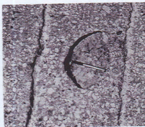
Fig. A.2.21.1-Small spall
