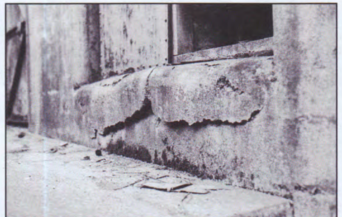
When corroded, metal expands to approximately ten times its original volume. The force is sufficient to break and detach surrounding concrete or masonry. Battery Tolles, Fort Worden, Washington.
