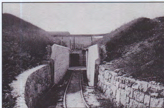
As the shift to concrete construction became more complete, masonry was relegated to a minor role as represented in this 1908 photograph of the retaining wall at the entry to Battery Butterfield, Fort H.G. Wright, New York.
