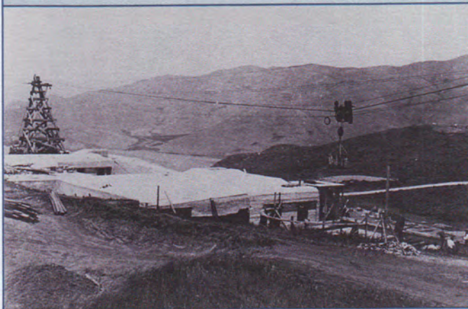
Figure 2. Construction of Battery Mendell, ca. 1902. Note the tramway erected to bring concrete plant to the cliff top site from a batching plant at the north end of the beach. Note the farm at the left center background—leased by a family of long-time dairymen of Portuguese decent.
