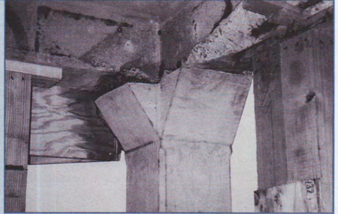
Figure 8. The repaired support pillar convincingly recreates the complex chamfers and cornices of the original.
