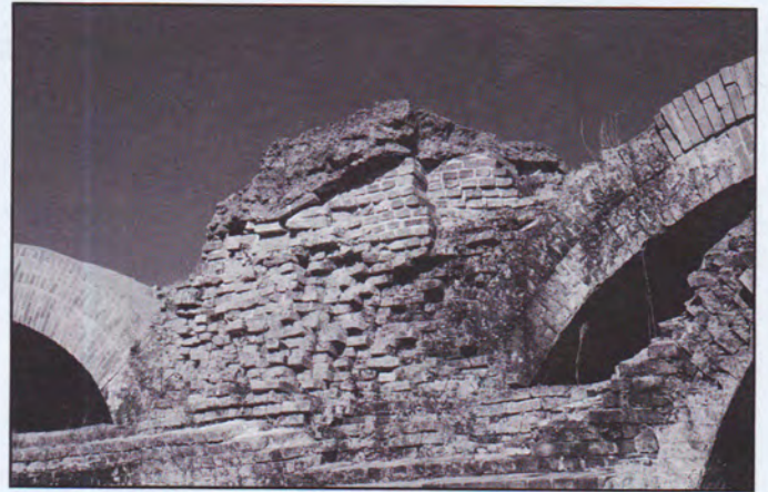
Loose in-fill between the vaults of masonry fortifications provide an ample reservoir for water that can steadily percolate to the interior even in dry weather. Fort Pickens, Florida.
