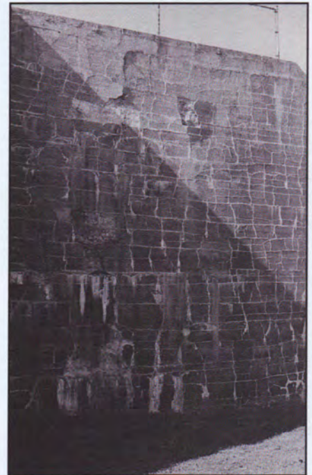
Vertical and horizontal cracks, efflorescence, and chloride deposits are characteristic of concrete fortifications of the early 1900s. Battery Harker, Fort Mott, New Jersey.
