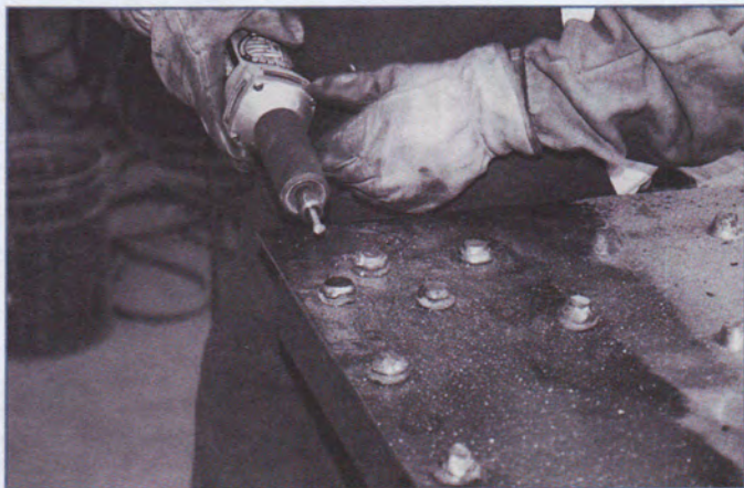
Figure 9. The two rivet elements were welded together and then shaped to the configuration of hot rivets.
