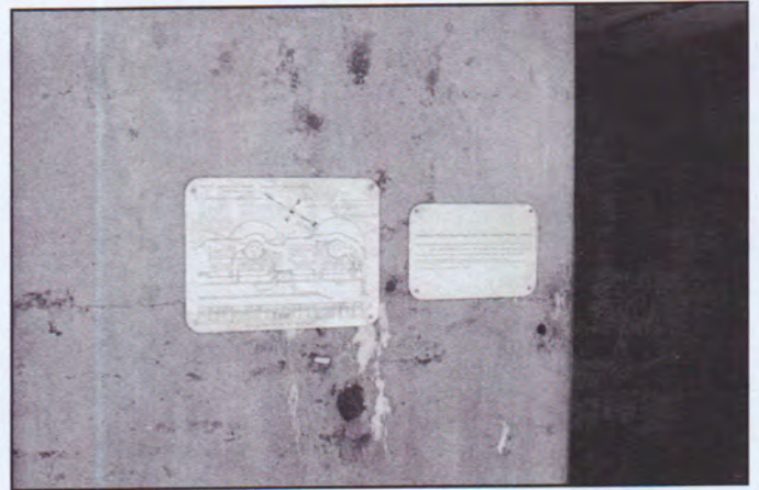
Signs bolted directly to a wall at Fort Casey. A preferred alternative would have been to attach the signs to non-intrusive brackets or freestanding bases.
