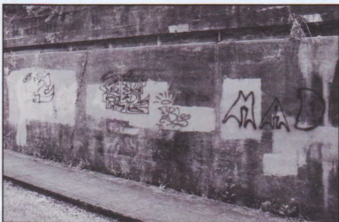
Painting over graffiti applied to concrete is a quick fix, and one that can help control its spread to previously unmarked areas of the structure. Battery Randol, Fort Worden, Washington.
