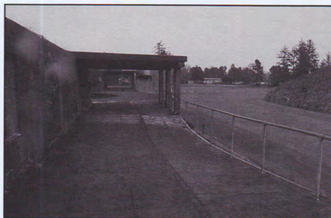
Sagging in a thin section platform extension. Fort Stevens, Oregon.
