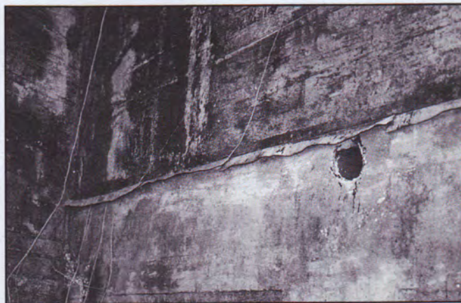
A sheet of non-ferrous metal acts as an impervious membrane between two concrete pours at Battery Pensacola, Fort Pickens, Florida.
