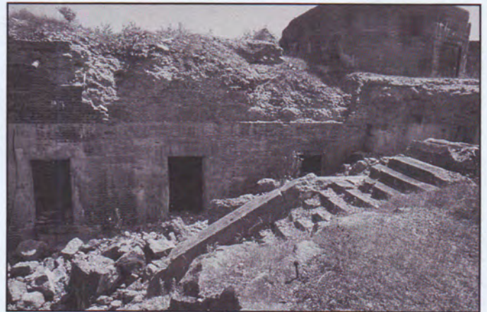
Extreme winter weather conditions have caused severe spalling in this battery at Halifax, Nova Scotia.
