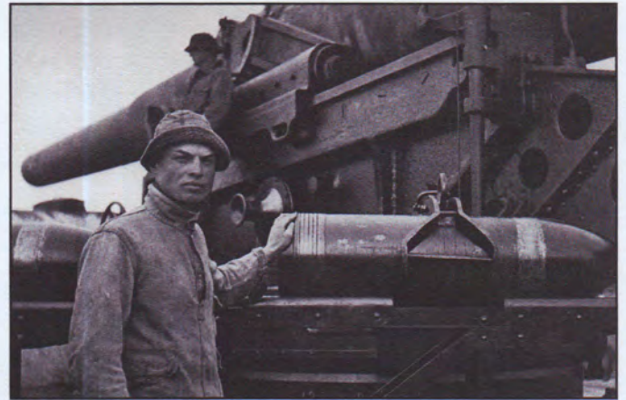
A half-ton projectile mid-way in its journey from the lower level of the emplacement to the breech of the gun. Battery Spenser, Fort Baker, San Francisco, California.
