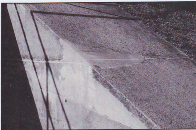
This view of a concrete repair at Battery Gregg was taken about five years after the work was completed. The patch is intact and appears to be well-bonded to the substrate.
