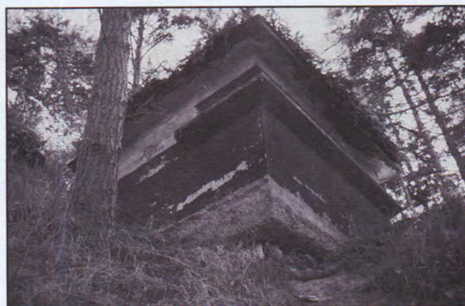
Bluff erosion can undermine structures and pose significant preservation challenges. Battery Kinzie Primary Station, Fort Worden, Washington.
