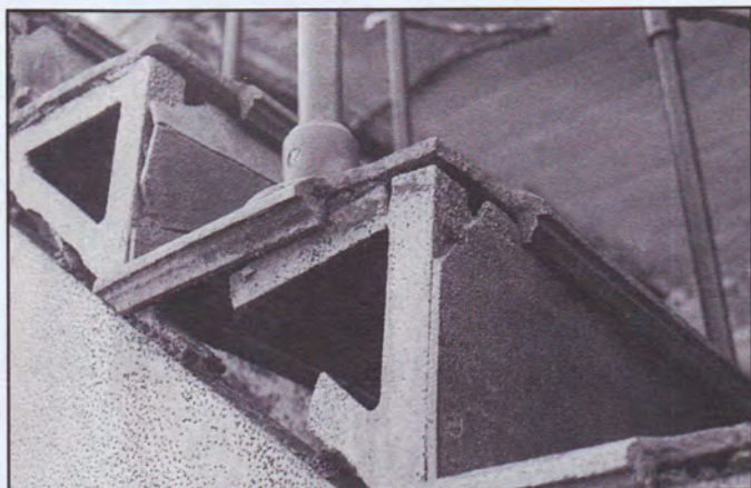
Repairing broken cast iron is difficult, especially if pieces are missing. Fixes include recasting a replacement section or fabricating a new section from appropriate substitute materials. Battery Harker, Fort Mott, New Jersey.
