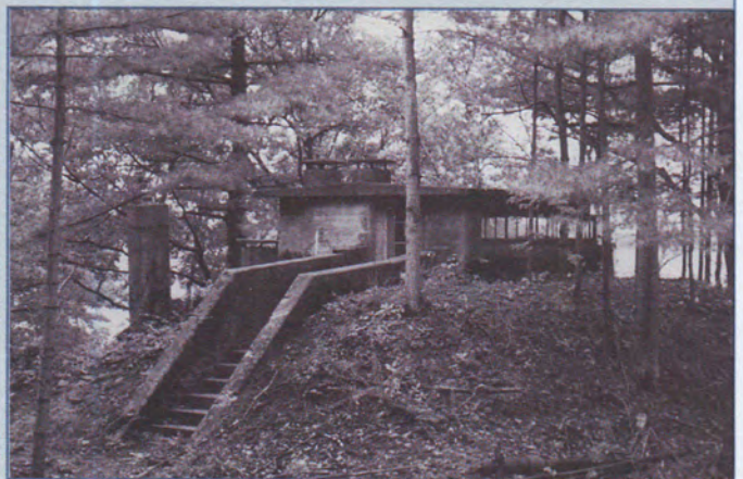
Figure 4. The 1920 range finder station built on top of the 1902 mining casemate. A coincidence range finder mounted in the station was to provide range data to the minefield defense battery located to the right.
