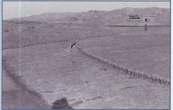
Figure 9. Looking north to BC station from the front of emplacement two, showing separation and subsidence of blast apron from the concrete mass of the remainder of the battery.
