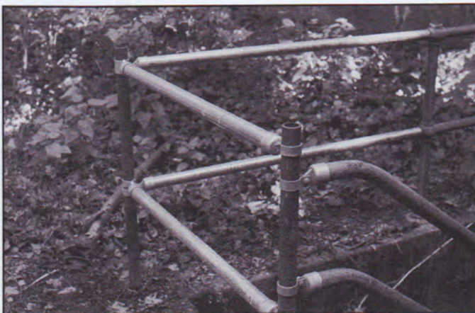
A simple and compatible replacement railing at Battery Thornburgh, Fort Ward. The railing clips to the original pipe rail stanchions.
