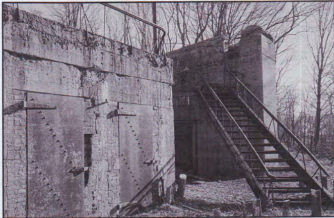
Plate steel, forged iron, galvanized iron, and structural steel shapes are all in evidence in this predominantly concrete fortification. Battery Richmond, Fort Wadsworth, New York.
