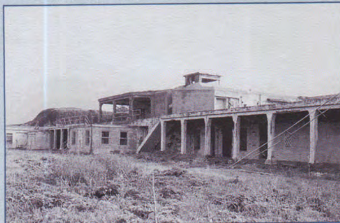
Figure 4. Deterioration such as spalling concrete and rusted railing is evident in this 1973 photograph taken shortly after Golden Gate National Recreation Area was established.
