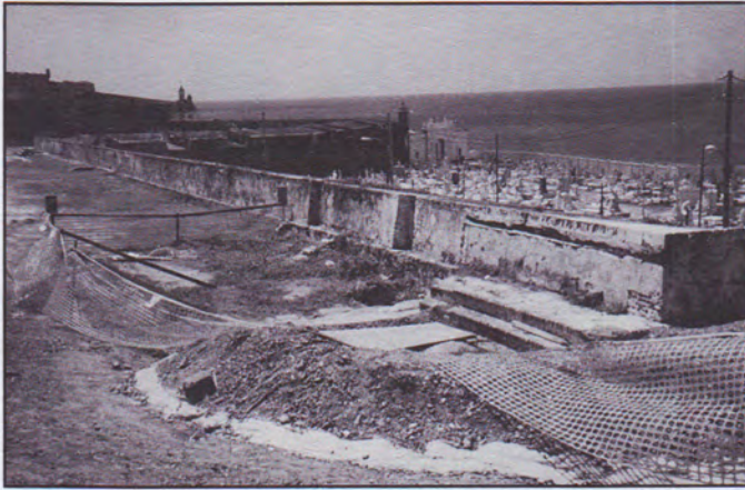
Above the area of the collapsed drainage tunnel, the terreplein has sunk and the stones of the firing steps along the parapet are beginning to drop away. City Walls, San Juan, Puerto Rico.
