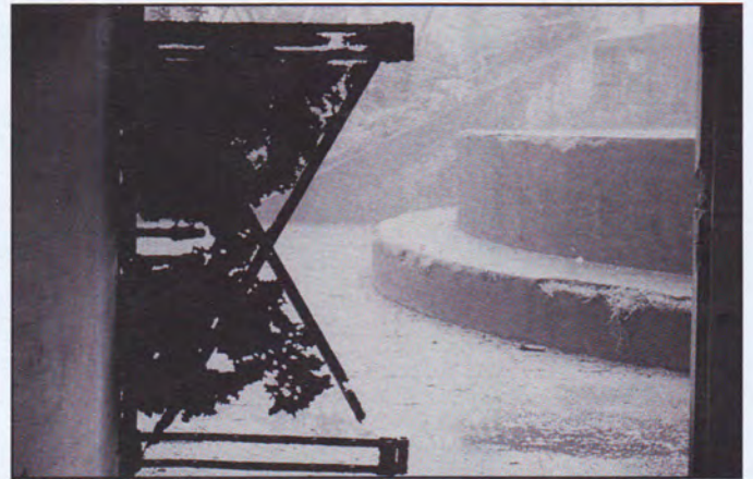
A wet climate and salt-laden fogs are ideal conditions for the rapid loss of ferrous metals, as suggested by this corroded door at Battery Harvey Allen, Fort Canby, Washington.
