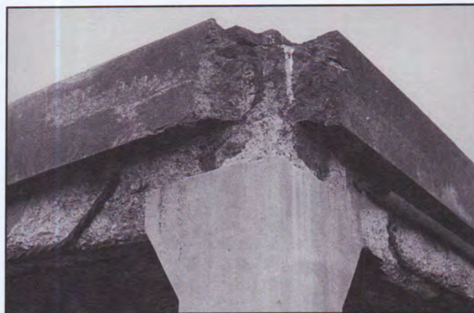
Broken concrete at Battery Mendell, Fort Barry, California. The likely cause is the expansive force of the corroded reinforcing steel visible in the photo.
