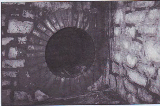
Both brick and stone masonry were used to form this ventilator opening in the otherwise concrete construction of Battery Thompson, Fort McKinley, Maine.
