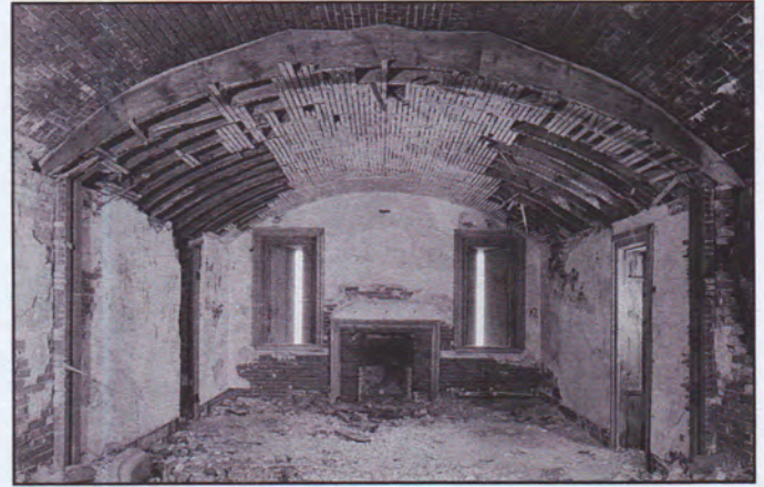
The edge of a sheet metal diversion membrane is visible above the lath and plaster ceiling of this casemate interior at Fort Gorges, Maine.
