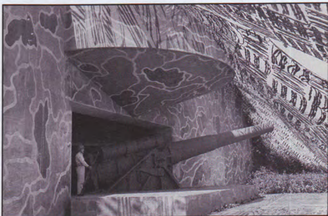
The camouflage is distinctive and clear in this 1943 photo, but such patterns can still be distinguished today, and would be lost in a program of comprehensive cleaning. Battery Reed, Fort Amezquita, Puerto Rico.
