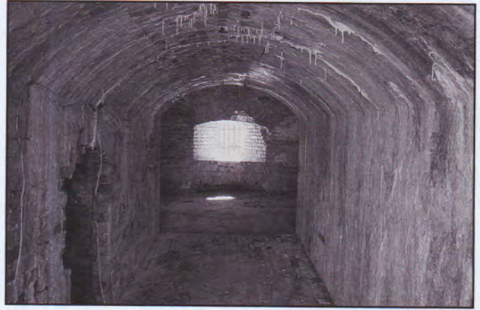
Stalactites and a heavy deposit of calcium carbonate coat the walls of this vault at Fort Macomb, Louisiana.
