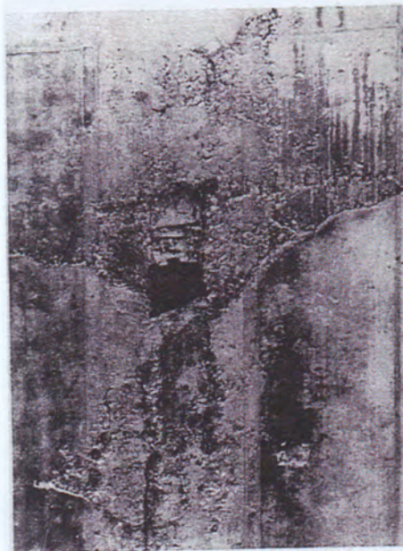
Fig. A.3.5—Cold joint
