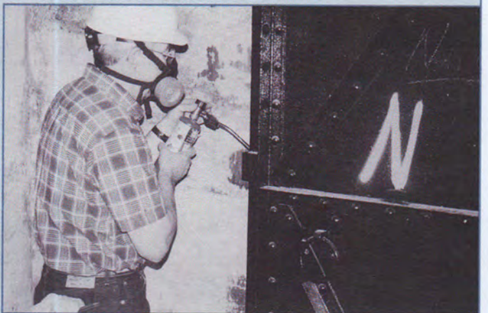
Figure 3. Using heat to loosen a frozen nut. Safety equipment was necessary because of the potential of lead paint hazard.
