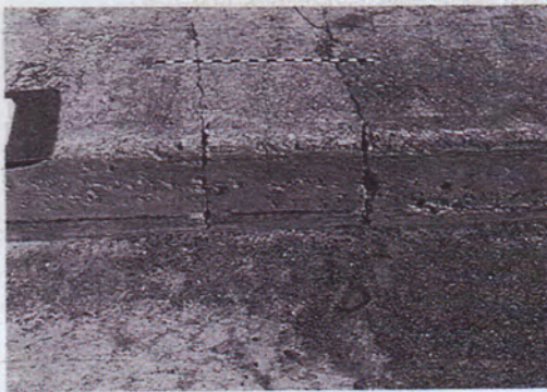
Fig. A.1.10-Transverse cracking (wide)
