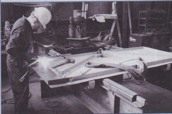
Figure 4. New steel plate being welded to an original door to replace the corroded section that has been removed.
