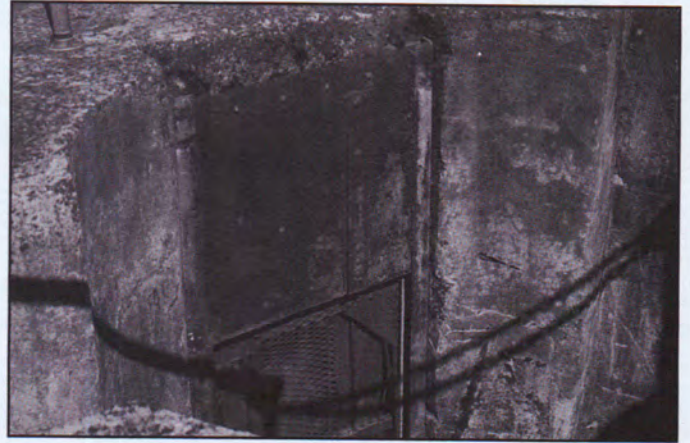
The historic resource should never be scavenged for materials. Doors taken from other locations have been cut and welded together to close this opening at Battery Mishler, Fort Stevens.
