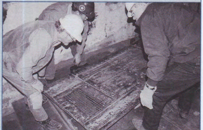
Figure 2. The door was lowered down to rest on wooden sleepers that had been positioned to receive it. The lighter color on the back of the door is the surviving layer of red lead.
