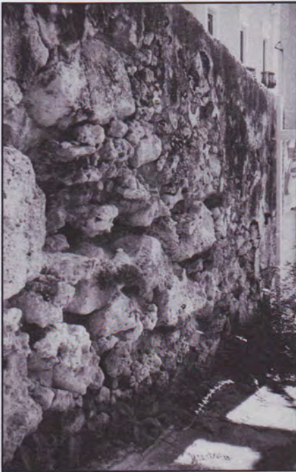
Critical lack of maintenance has led to advanced deterioration of the city walls in San Juan. The binder is all but gone, and only the weight of the stones hold them in place.
