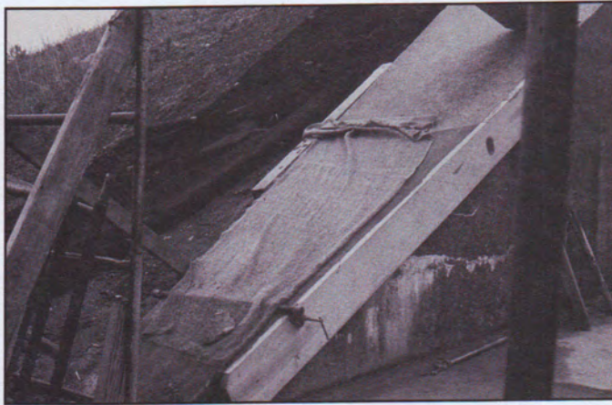
After new concrete was placed in the patch area, it was covered with burlap to encourage a better cure. Battery Gregg.
