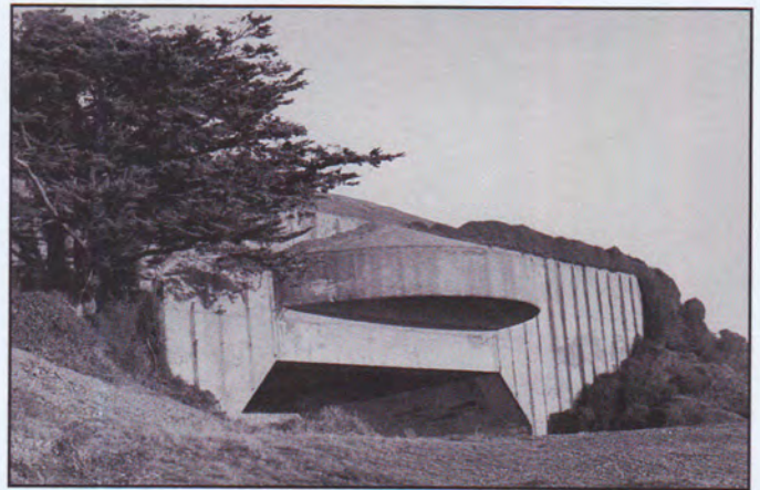
Heavy rust stains mark the exterior of Battery Townsley, Fort Cronkhite, California.
