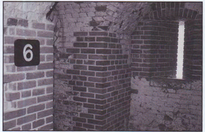
The restoration of this brickwork has been done in a manner that distinguishes the area of the repair while remaining compatible with the surrounding original masonry. Fort Barrancas, Florida.
