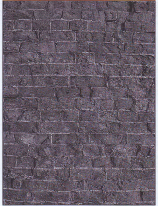
Exterior wall surface in poor condition—note use of non-lime based mortar for finish pointing of joints also eroded face of bricks.
