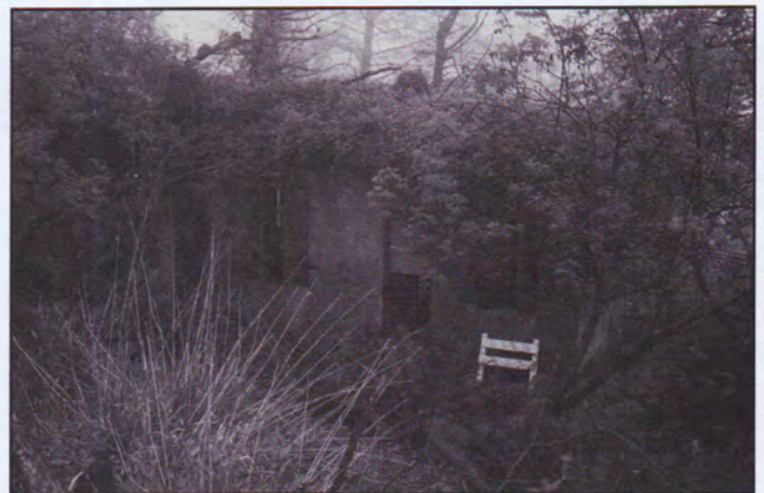
Uncontrolled plant growth can lead to the rapid deterioration of wood-frame structures that are also part of many fortifications. Fire Control Dormitory, Fort Canby, Washington.
