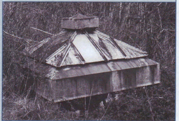
Evidence of skilled workmanship. Galvanized iron ventilator, Fort Columbia.
