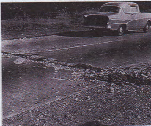
Fig. A.2-Disintegration
