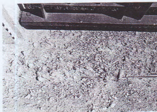
Fig. A.2.20.4b-Close-up scaling (very severe)
