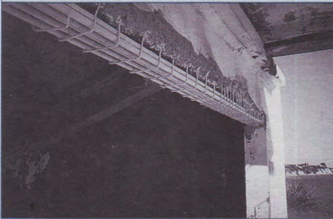
Figure 6. Reinforcing steel primed prior to plastering, Fort Takapuna.
