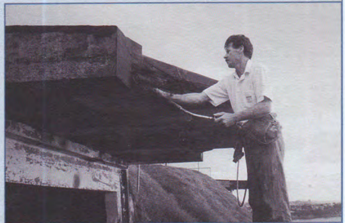
Figure 4. Applying waterproof membrane to emplacement roofs, North Head.
