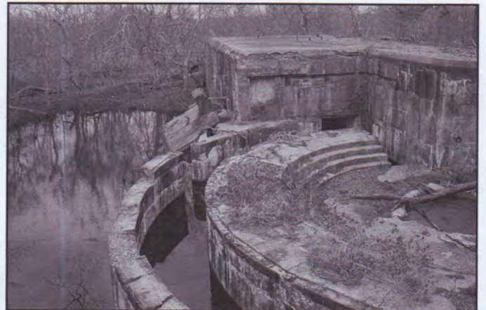
Poor construction sites become poor historic sites, as demonstrated by the persistent high water table at Battery Forse, Fort St. Phillip, Louisiana.
