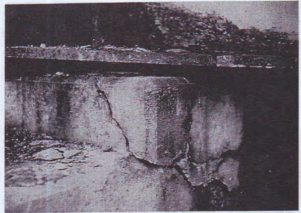
Fig. A.1.4-Diagonal cracks
