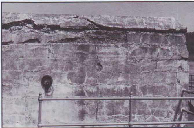
Long regarded as the result of freeze/thaw cycles, this linear spall appears to be more the product of poorly mixed and placed concrete. Fort Casey, Washington.
