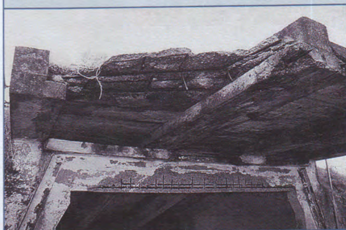
Figure 2. Spalling concrete, four-inch emplacement, North Head.
