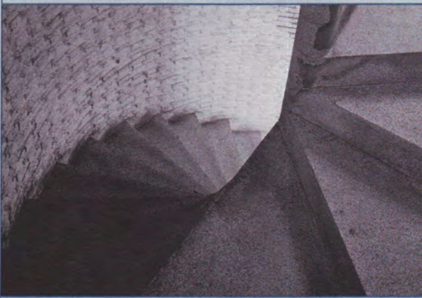
Evidence of skilled workmanship. Spiral granite stair, Fort Point.
