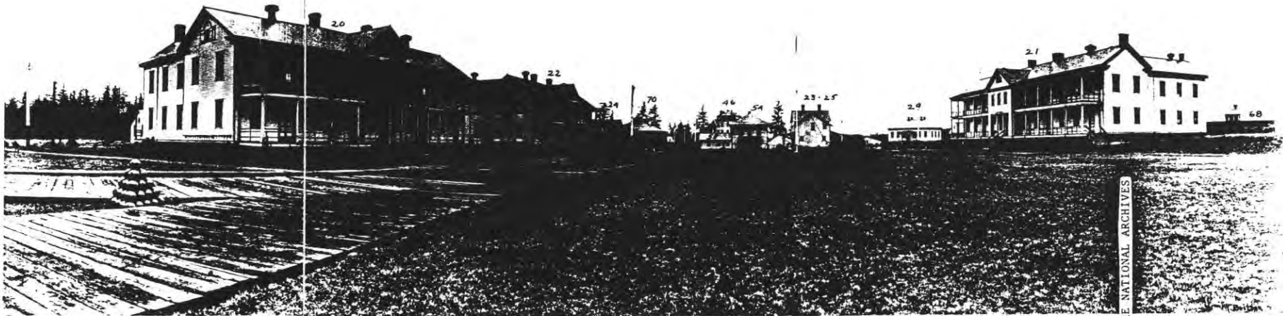
View from Headquarters, looking North.
