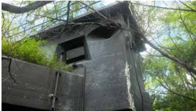
Indicator Display at Battery Hasbrouck
