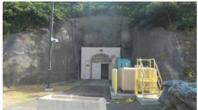
Rear Entrance to Battery 407
