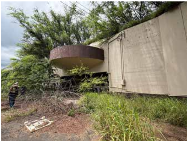
Battery Closson emplacement
