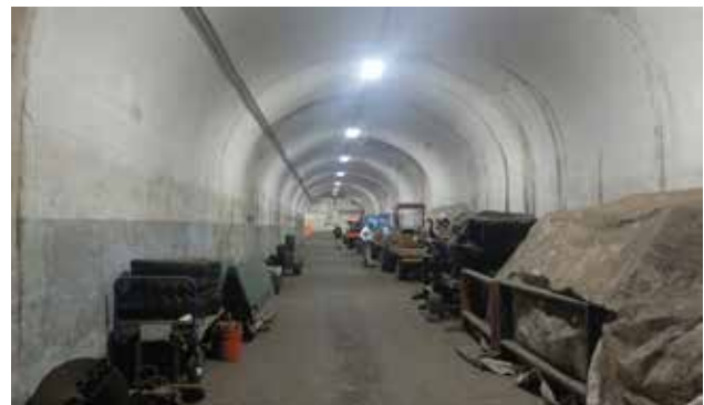
Battery 304 lateral tunnel
