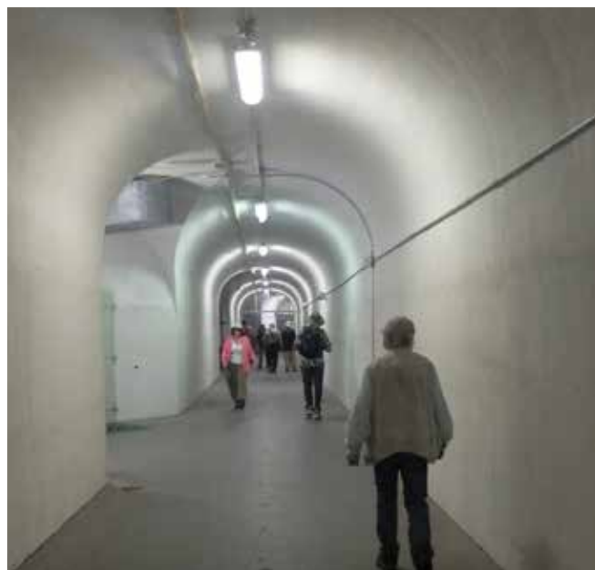
Battery 407 interior corridor
