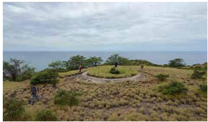
Battery Arizona's filled in turret ring
