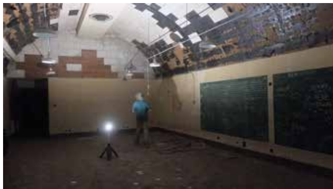
Battery Arizona Plotting Room
