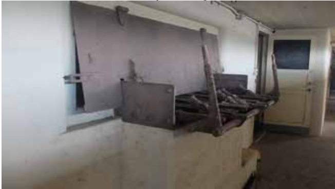
Shell receiving tables at Battery Selfridge
