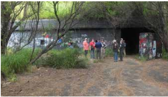
Battery Hasbrouck Pit A
