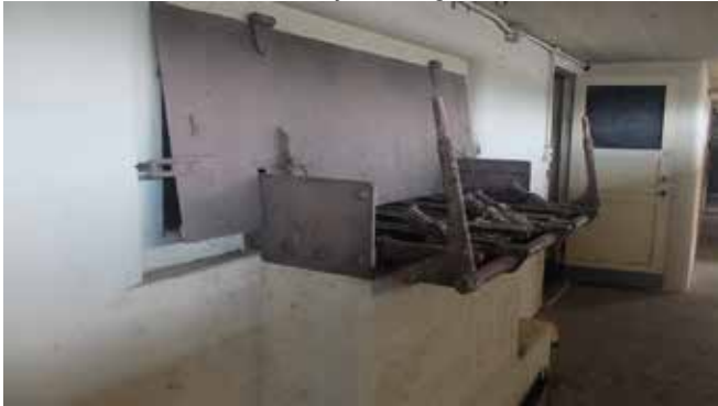
Shell receiving tables at Battery Selfridge
