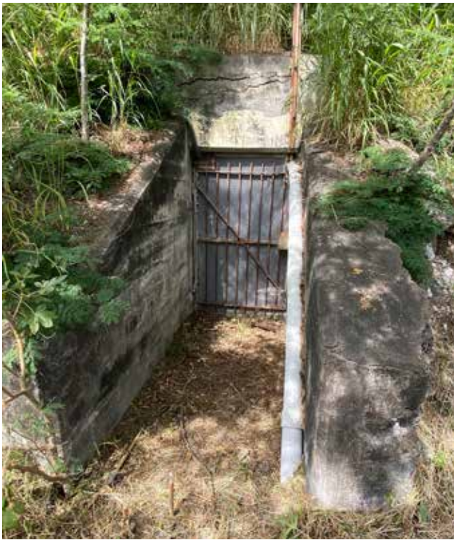
Entrance to Battery Dodge
