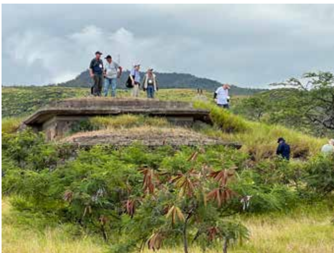
Battery Arizona Battery Commander's Station
