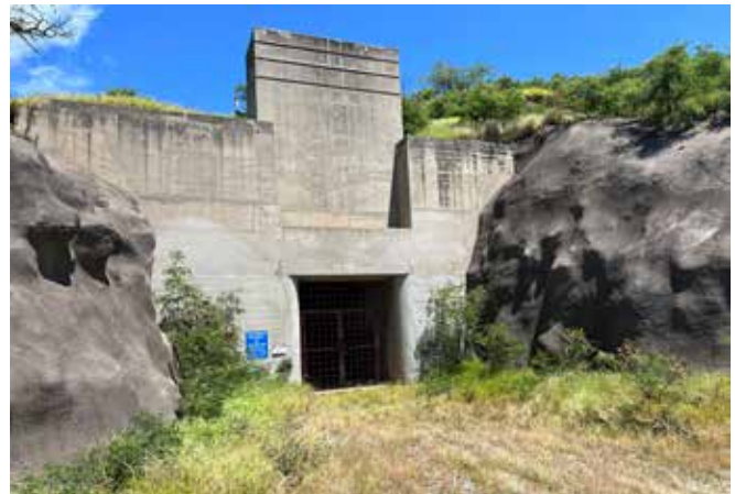
Battery Arizona Entrance Portal
