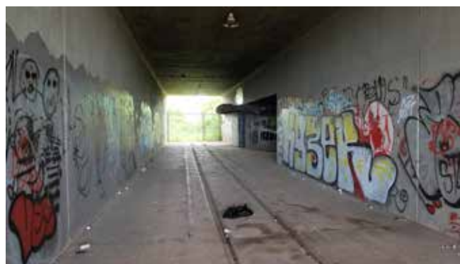
Inside one of the emplacements of Battery Hatch
