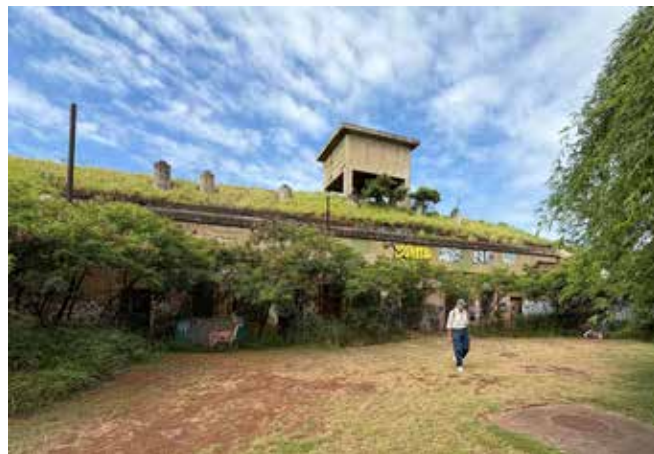
The plotting room and battery commander's station of Battery Hatch
