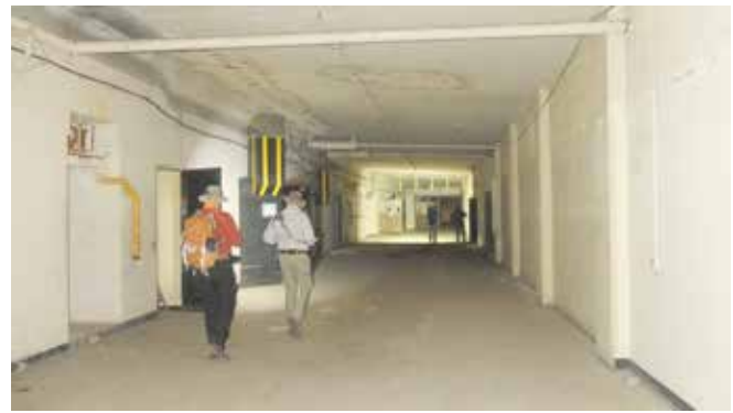
Main Corridor in Battery Closson
