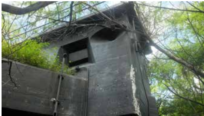
Indicator Display at Battery Hasbrouck
