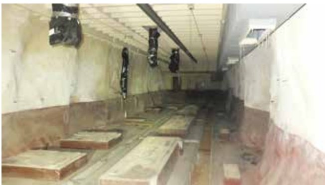
Battery Pennsylvania Power Room
