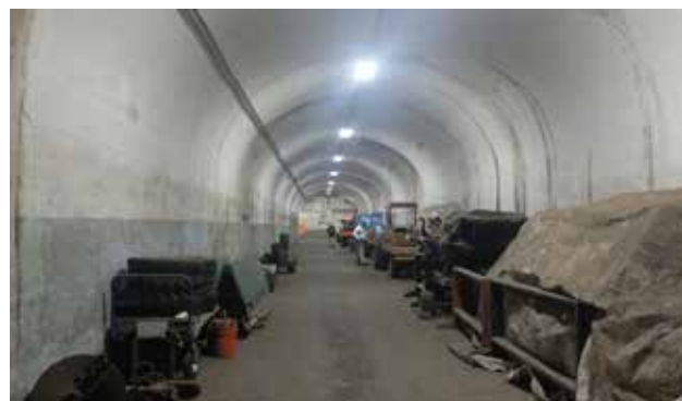
Battery 304 lateral tunnel
