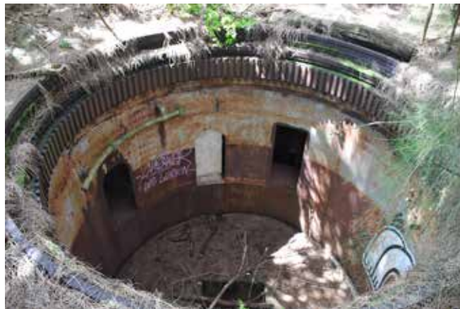
Recent photo of one of the 8-inch Navy mount gun well for Battery Kirkpatrick, Oahu, Hawaii
