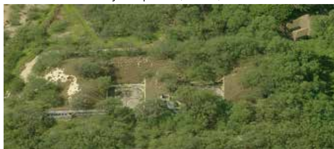
Recent photo of Battery Hasbrook, Fort Kamehameha, Oahu, Hawaii.
