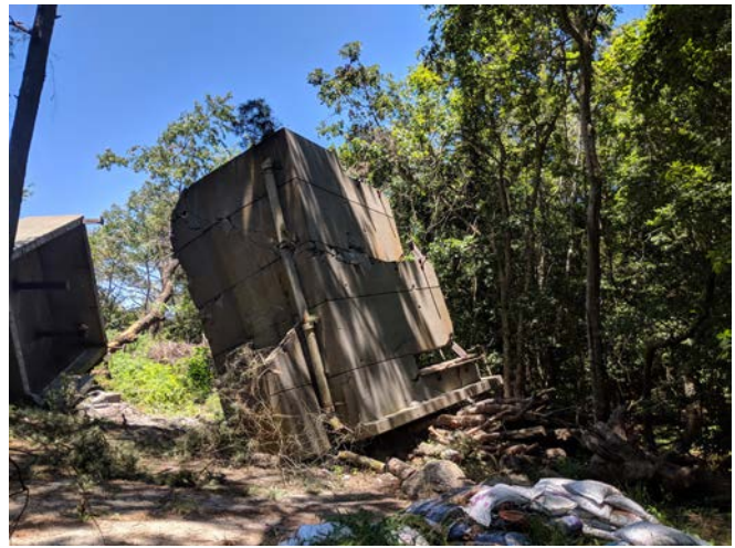
Cheapside Fire Control Tower today. Tower has been toppled with concrete station broken into two parts with the upper station upside down. (McGovern Collection)
