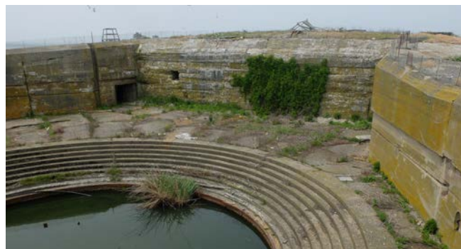
Recent view of Battery Davis (16-inch DC), looking at the loading platform with the gun well full of water and entrance to the magazines near the back wall. McGovern Collection.
