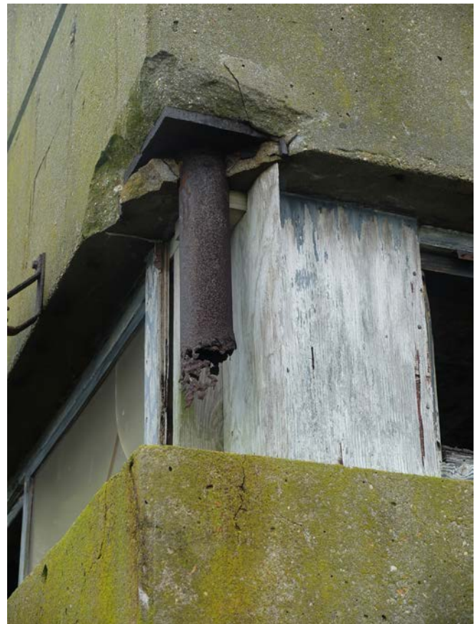
Closeup of the rusting steel supports for the observation window at the mine station at Fort Wool, VA. This problem has become widespread with battery commanders, CRF, and fire control stations. Without replacement supports these structures will collapse. (McGovern Collection)
