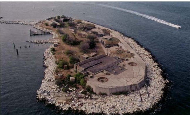
Fort Wool on Rip Raps Island, Hampton, VA. WW2 Battery Gates (two 6-inch shielded BC) in the foreground with the two Endicott-Taft 6-inch disappearing gun batteries in the middle and the remaining 3 rd -System casemates in the background with the two 3-inch rapid-fire batteries. (McGovern Collection)
