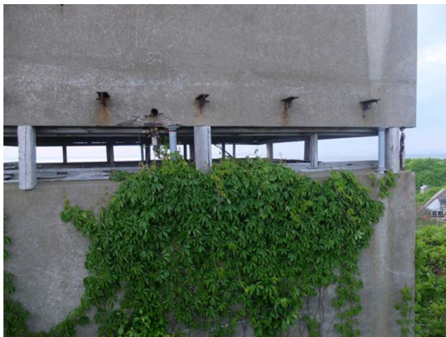
Fire control tower I-E showing temporary wooden blocks and steel pipes supporting the ceiling. Original steel posts have rusted away. McGovern Collection.
