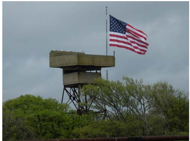
Battery Gates' BC station is a concrete station with CRF on the roof, on a steel tower at Fort Wool. The roof is hinging forward as the steel supports on the observation windows is rusting away. (McGovern Collection)
