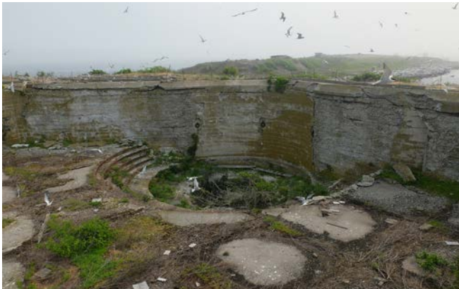
Recent view of Battery Palmer's 12-inch DC loading platform. Note extensive spalling of parapet walls. McGovern Collection.
