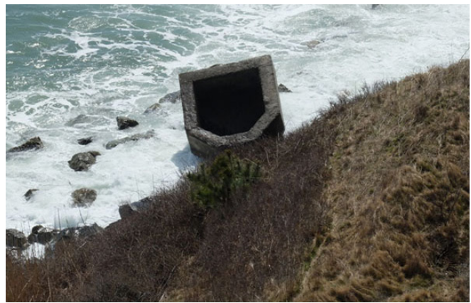
Montauk Point dug-in FC station tumbled onto the beach
