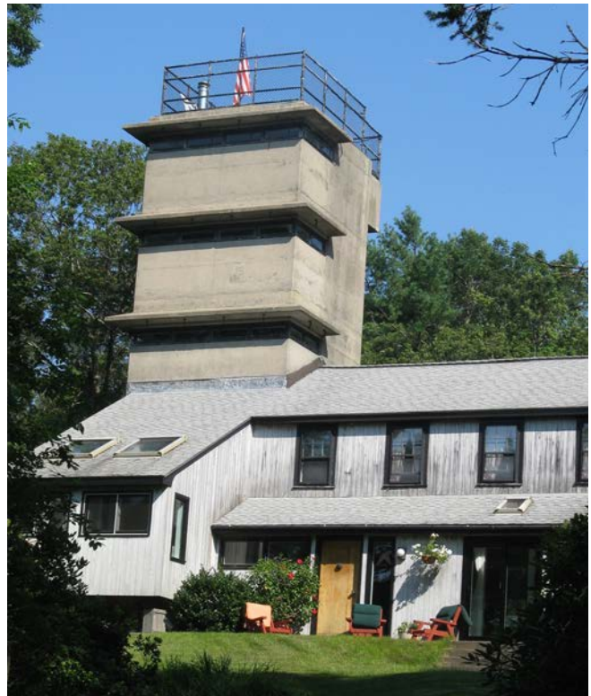
Coolidge Point fire control
