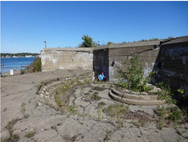
Fort Constitution Battery Farnsworth gun platform
