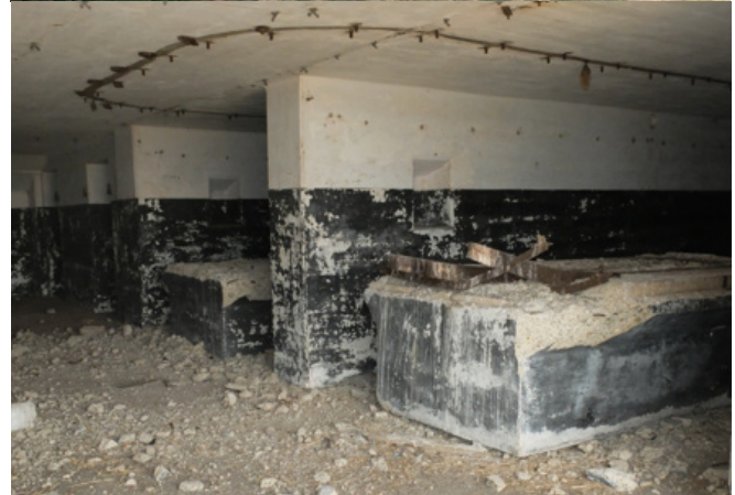
Battery Webb – 2 x 14-inch/DC – Fort Randolph – Shell tables
