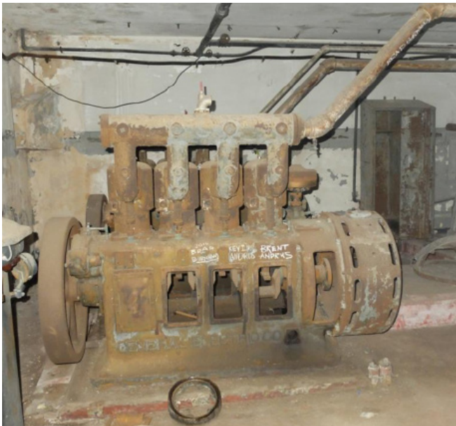
Battery Warren – 2 x 14-inch/DC – Fort Grant – 25kW motor generators
