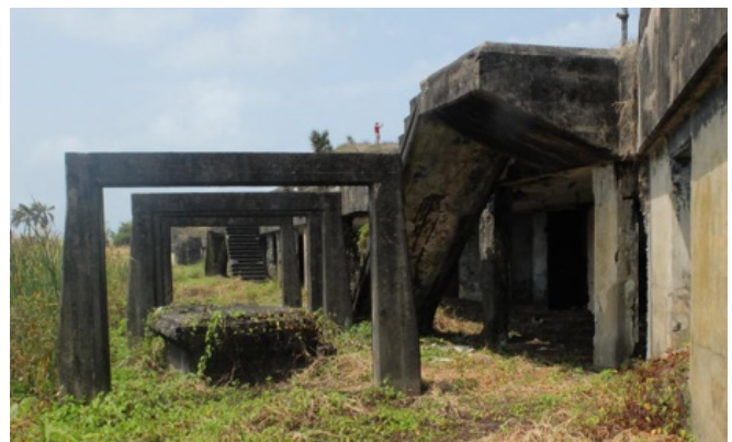
Battery Webb – 2 x 14-inch/DC – Fort Randolph – 14-inch railway shell table and overhead rail supports
