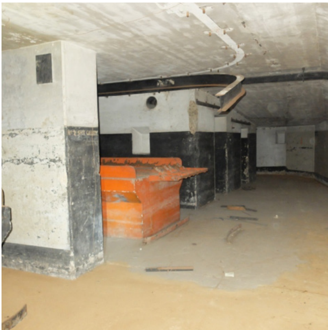
Battery Buell – 2 x 14-inch/DC – Fort Grant shell table in magazine
