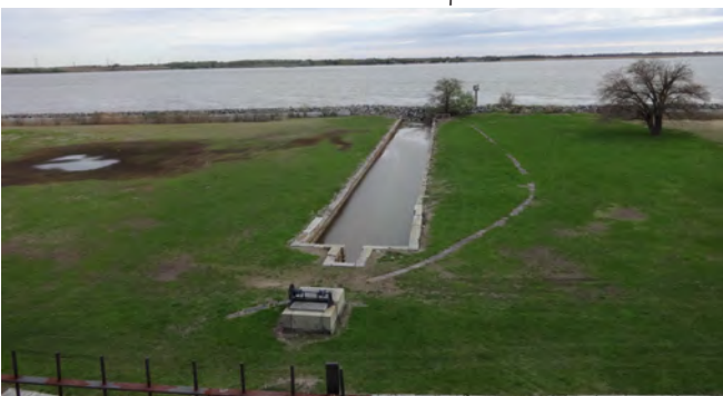
Tide sluice and gate for Fort Delaware's moat
