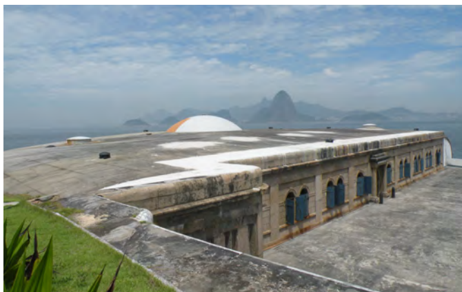
Gorge of Imbuhy fort. The steel shutters in the windows are provided with rifle loopholes for local defense.
