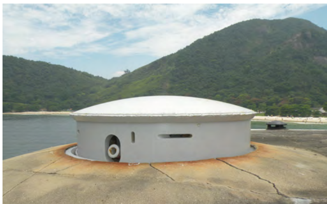
Partially raised retractile turret for one Krupp 75 mm L/25 local defense gun. The gun is in the rest position.
