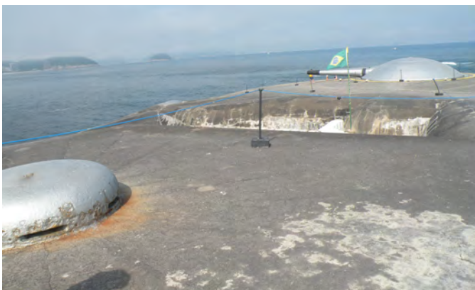
Observation cloche, with the main cupola of Copacabana (two 305 mm L/40 krupp guns) in the background.
