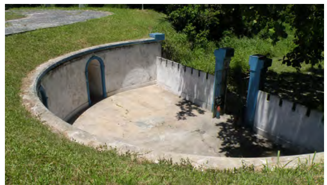
Central hall, with galleries leading to the individual guns. In these galleries there are rooms to store ready-use ammunition.
