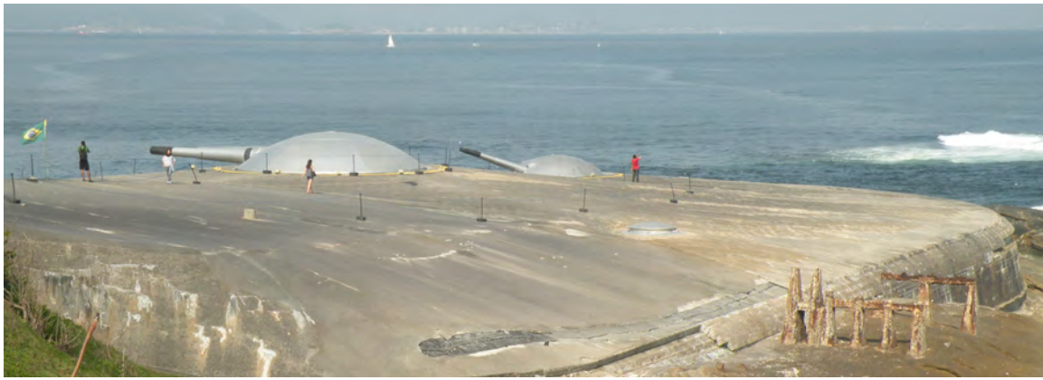
Top of Copacabana fort with its two gun cupolas. It is also possible to see the top of one of the two 75 mm L/25 retractile turrets of the fort.
