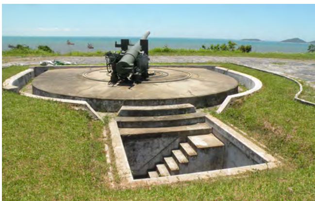
Forte Marchel Hermes Gun position, showing the stairway leading to the ready-use ammunition magazine
