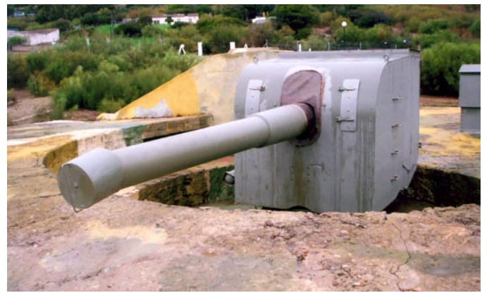
14. A "W" gun with its cap to protect the gun barrel. Note the cracking of the concrete around the gun.
