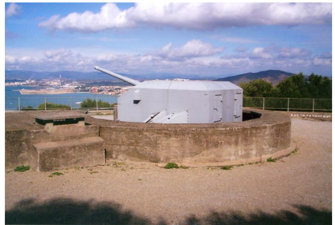
23. Princess Anne's No. 3 Gun showing the ammunition ventilation outlet.
