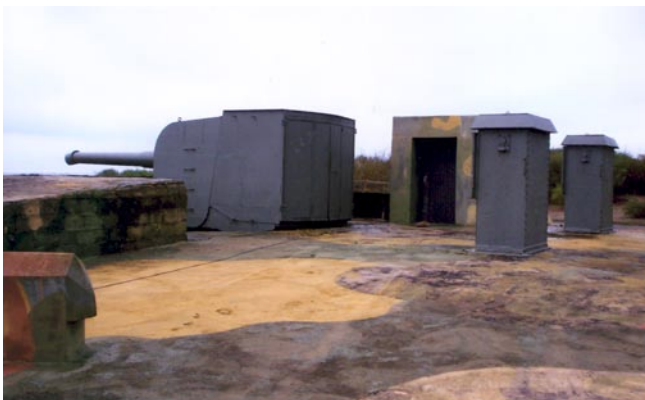
13. A "W" gun position showing the extensive concrete apron around some of these guns. The concrete has received camouflage paint.
