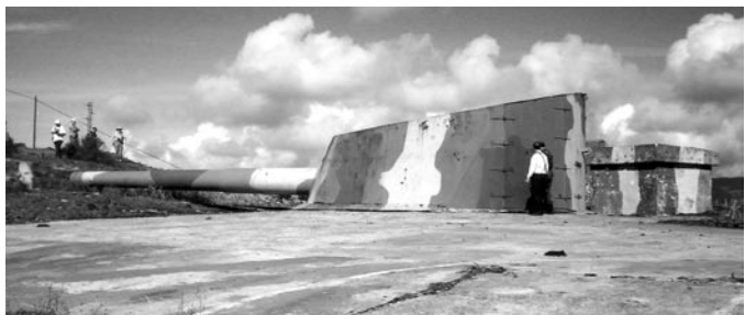
5. Side view of Battery Cascabel. The flaring skirt around the base of the shield carries rainwater away from the turret.
