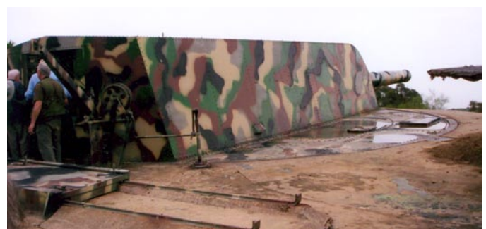
5. A close-up of the turret and the plate it rides on around the concrete apron. The standing water on the metal ring is from a recent shower.
