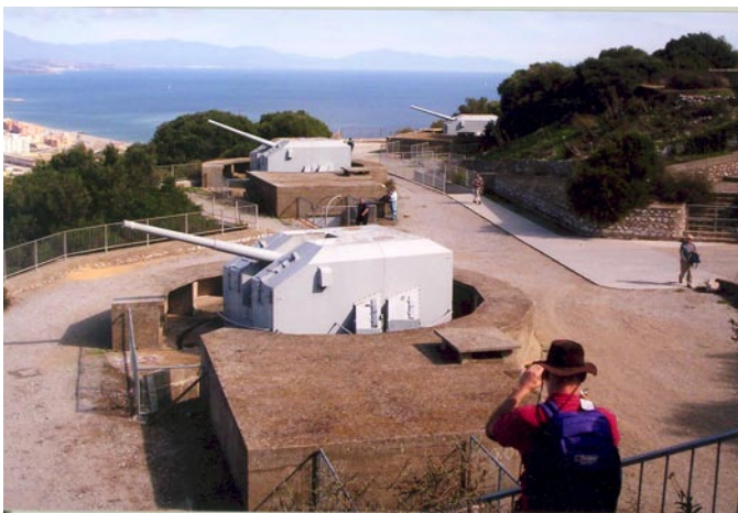
20. Princess Anne's Battery. The closest gun is No. 3. Note the concrete shelf running around the guns. The magazine for each gun is in the concrete house to the left of the gun
