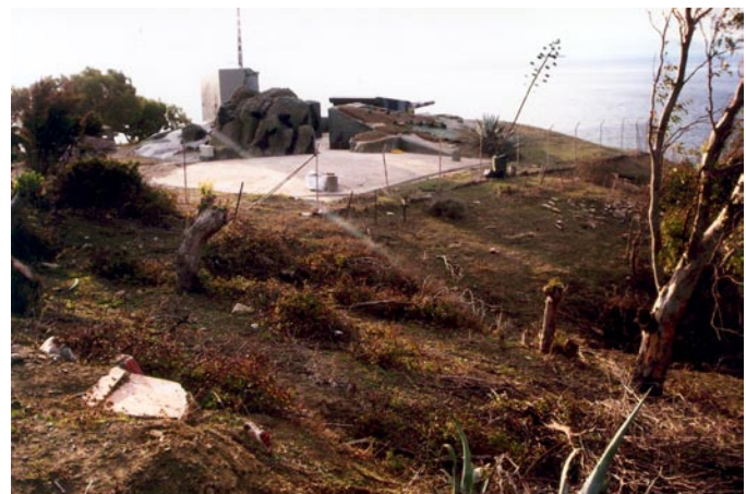
20. The 152.4 mm "V" gun positions from the barracks area. This gun came from the cruiser Miguel de Cervantes . The concrete support structures have been formed to look like rock.
