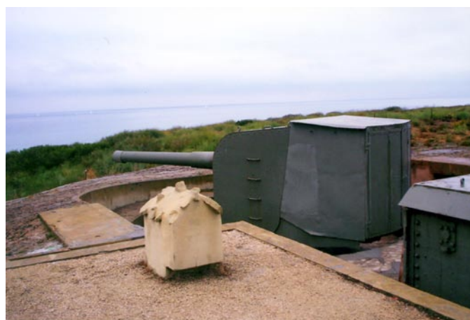
9. A companion "W" gun with protective cap on the end of the barrel and the porch on the rear of the gun to protect the breech. The gun sits in a slight gun pit with a concrete apron extending beyond the gun position.
