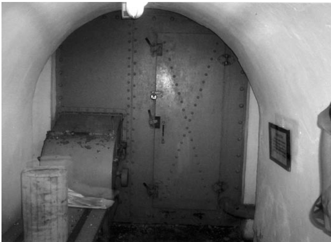
26. The Camposoto Battery powder magazine handling door and powder distribution tray. The powder bags were passed into the handling area via the metal container on the right. When the lid was lifted to access the powder bag, a shutter dropped, sealing off the powder-handling area from the powder magazine. When the lid closed, a shutter rose and the powder magazine could insert another powder charge into the handling tray.
