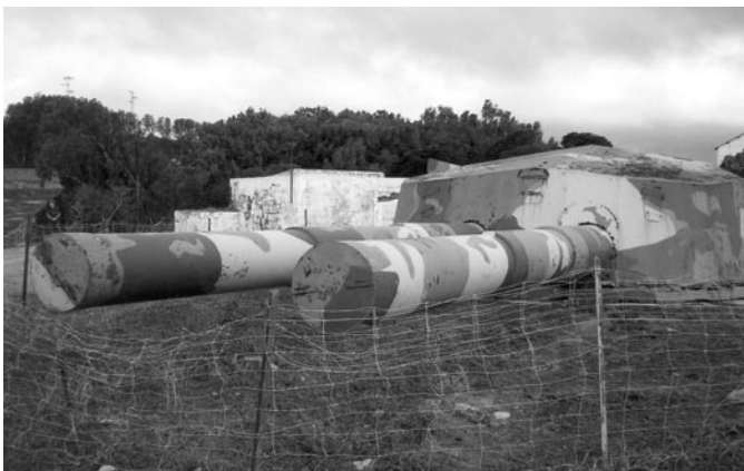
11. Battery El Vigia. The gun caps that protect the barrels extend 100 mm over the barrel, with camouflage paint matching the barrel. A rust streak on the left barrel marks where the cap ends.
