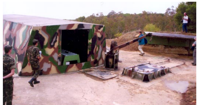
4. The rear of one of the 381 mm guns showing the opening through which the powder charges are passed into the turret. The crane and the trap opening are for loading shells into the shell magazine.
