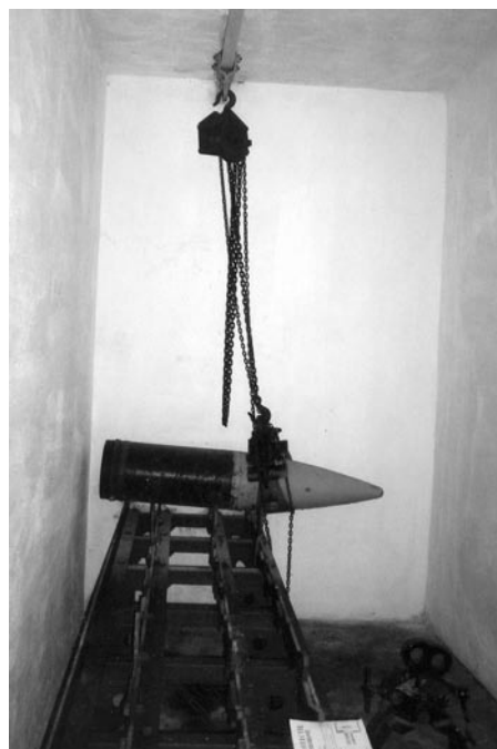
21. One of the shell-holding passageways within the Camposoto Battery, with a demonstration round on the shell rack. The shell was picked up by a clamp hanging from a monorail. Manpower moved this to the shell hoist opposite the powder room. Each shell rack held eight shells and there are ten shell-holding alcoves.
