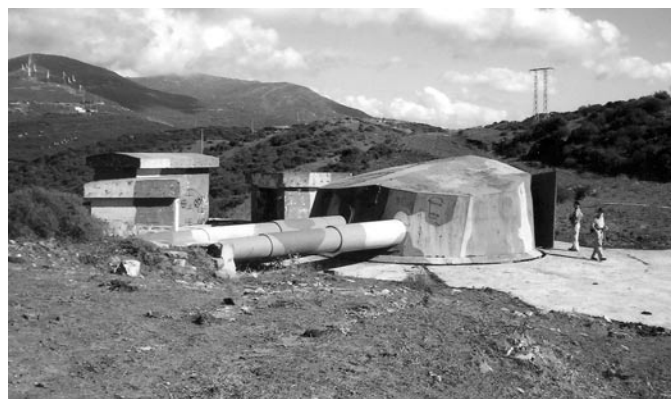
1. Battery Cascabel, one of two twin 305 mm/50 gun turrets installed at Tarifa in 1941. No longer active, it is in excellent condition. Support structures in the background provide access to the underground magazine and support rooms.
