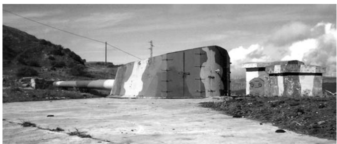
2. One has to wonder about the effectiveness of the camouflage paint at Battery Cascabel with the large white blast apron in front of the gun. The metal box behind the turret was used to replenish the magazine with shells and propellant.
