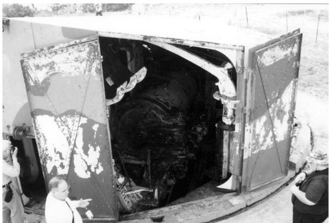
14. Battery El Vigia from above. The gun is covered in heavy Cosmoline to preserve it. Note the thin metal shield.
