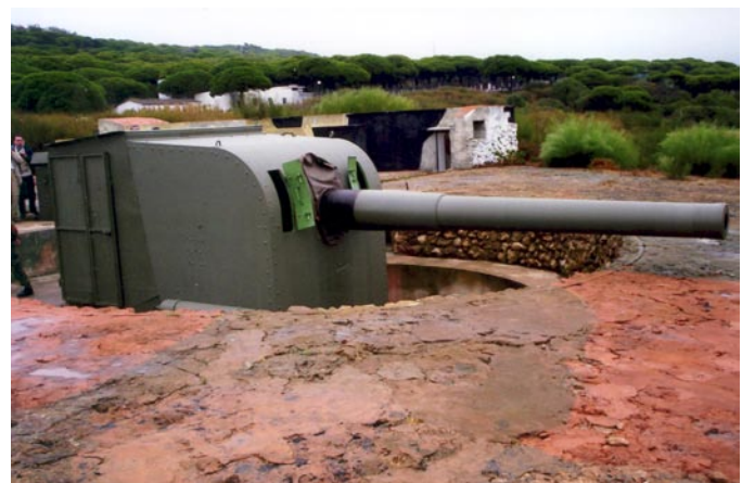
15. A side view of a "W" gun. The concrete building to the right of the gun, rear of photo, provides access to the magazine. The doorway at the right is to a ground-level hallway that leads to steps down to the magazine.
