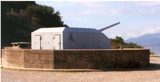
21. Princess Anne's No. 1 Gun showing the concrete wall around it. The magazine is to the left of the gun, underneath the ventilation structure.
