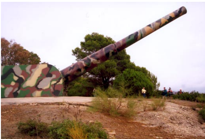
1. One of the three 381/45 guns at Battery Paloma Alta, raised for maximum range. The guns at the battery all had camouflage paint. A small concrete blast apron that did not extend to the length of the gun barrel surrounded the turret.
