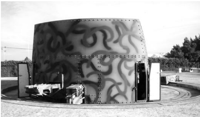
25. The rear of the Camposoto Battery. Note the thin shield and the depression that the gun sits in, unlike the guns at Tarifa.
