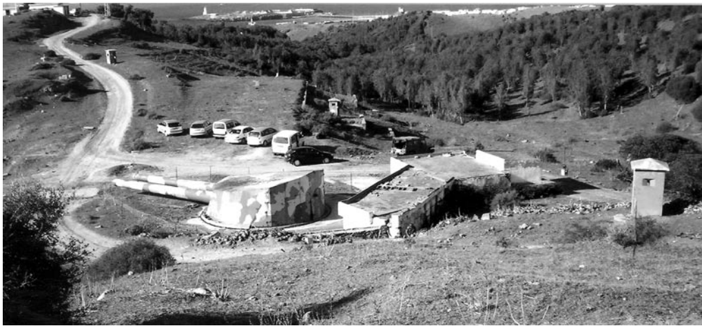
9. Battery El Vigia, one of two twin 305 mm/50 coast defense batteries built at Tarifa in 1941. The support structures at this battery are considerably different from those at Battery Cascabel, and the battery lacks a blast apron.
