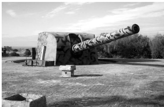
18. The 305 mm gun of the Camposoto Battery at almost sea level. Beneath the gun is an extensive bunker. Due to the greener vegetation near Cadiz, the gun's camouflage is green, not brown like at Tarifa. The gun sits in a shallow depression with a 360-degree blast apron, in theory capable of defending Cadiz against land attack.
