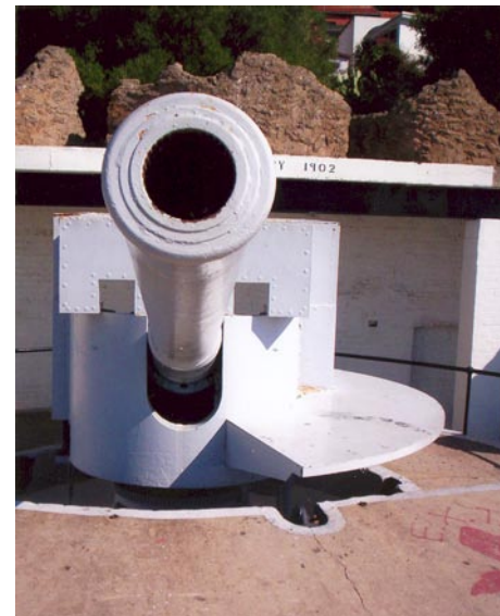
18. Devil's Gap No. 2 Gun. Note the metal ring extension, part of the original gun mount rendered useless by the new gun shield.
