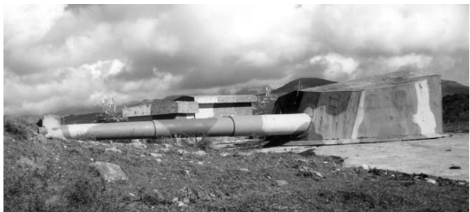
3. Battery Cascabel's guns swung 90 degrees to the right of their field of fire, barely clearing a concrete wall. In theory, with the guns in this position no one could toss an explosive charge down the gun barrel.
