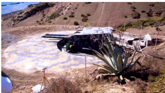
21. A "V" gun position showing the extensive concrete blast apron around it. The gun and apron have had camouflage paint applied.
