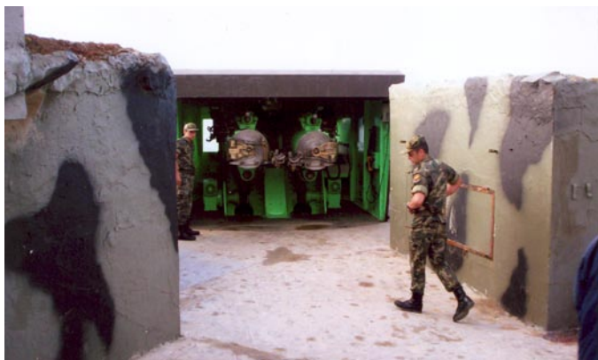
24. The entryway into the "V" gun position. The camouflage paint shows up on the horizontal structures. Note that the roofs are rough, to simulate ground.
