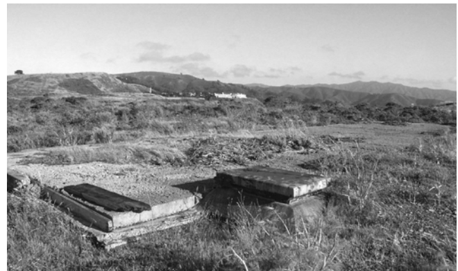
Concrete slab atop one of the Nike SF-51 magazine elevator doors, and crew escape hatch.
