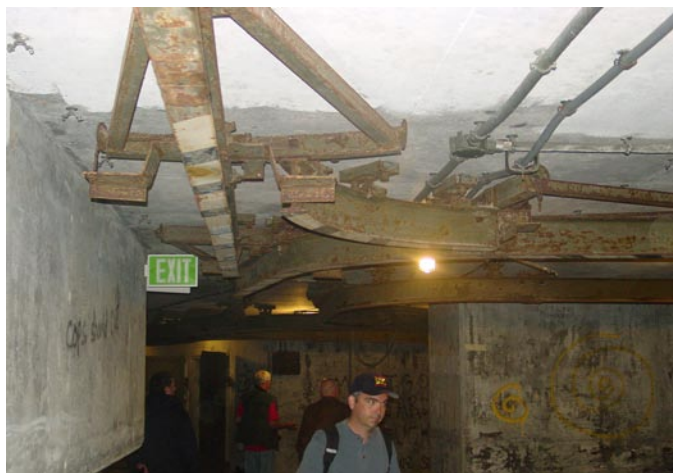
Overhead trolley rails of Battery Townsley, Fort Cronkhite
