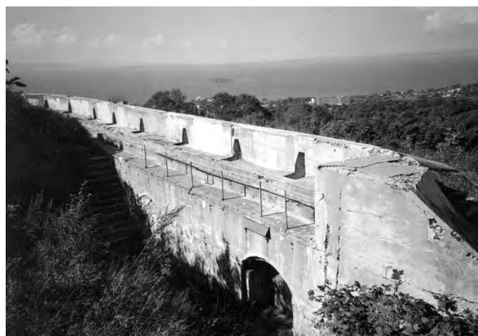
Concrete rifle parapet at Fort No. 7. Note the niches along the firing platform for rifleman shelters, and the doorway below for entry into galleries running under the parapet.
