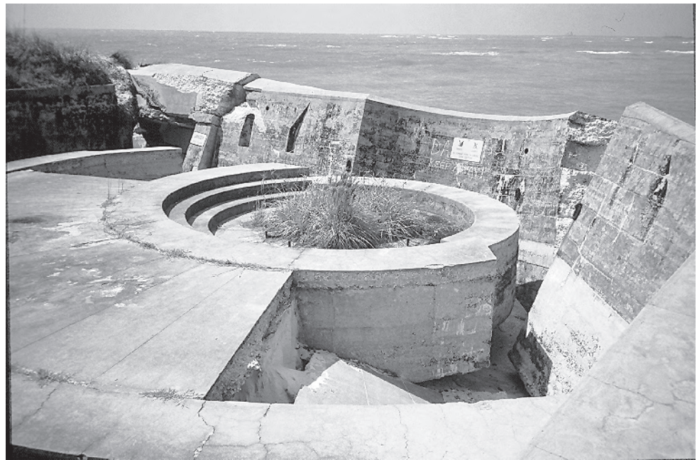
Erosion damage at Fort Dade: the fallen parapet of Battery Guy Howard.
