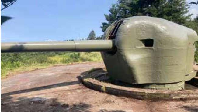
6-inch shielded BC at Battery #282 at Fort MacAndrews
