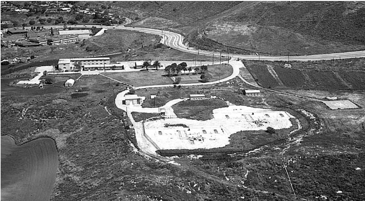
Nike Launch site LA-55L at Point Vicente on the Palos Verdes Peninsula
