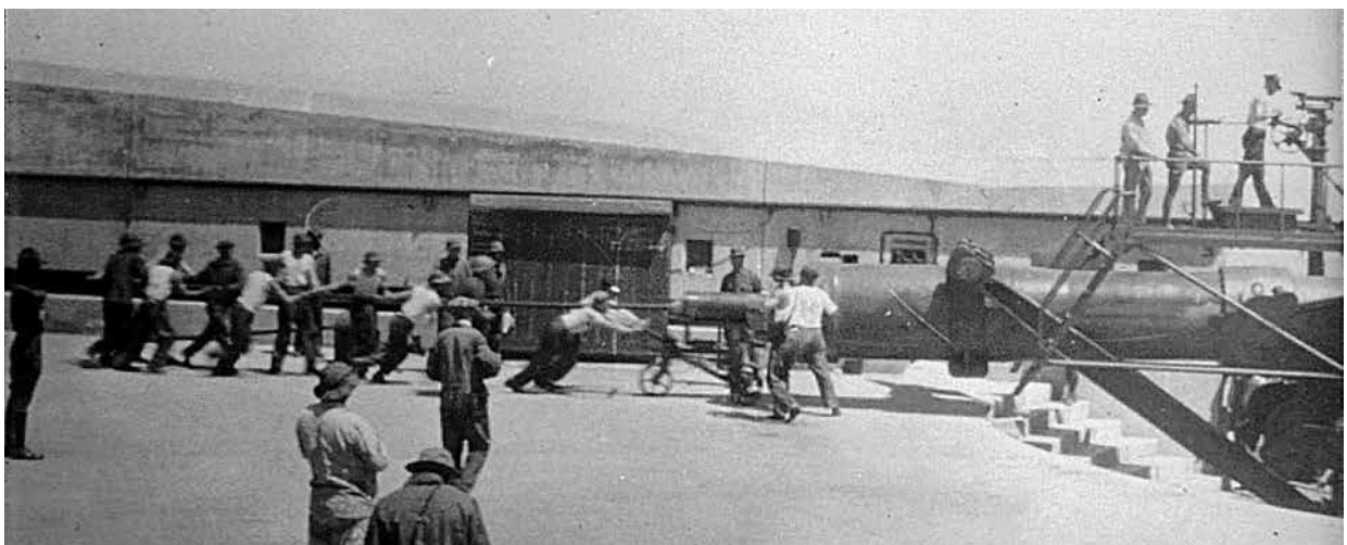
Battery Osgood, 1920s (Fort MacArthur Museum Collection)
