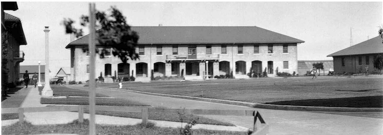
Barracks, Fort MacArthur, 1923 (George Ruhlen Collection, Fort MacArthur Museum)
