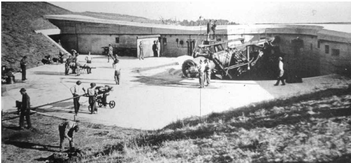
Battery Osgood, 1920s (Fort MacArthur Museum Collection)
