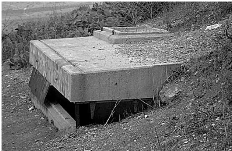
Base End Station, Point Vicente 1994 (photo by Mark Berhow)
