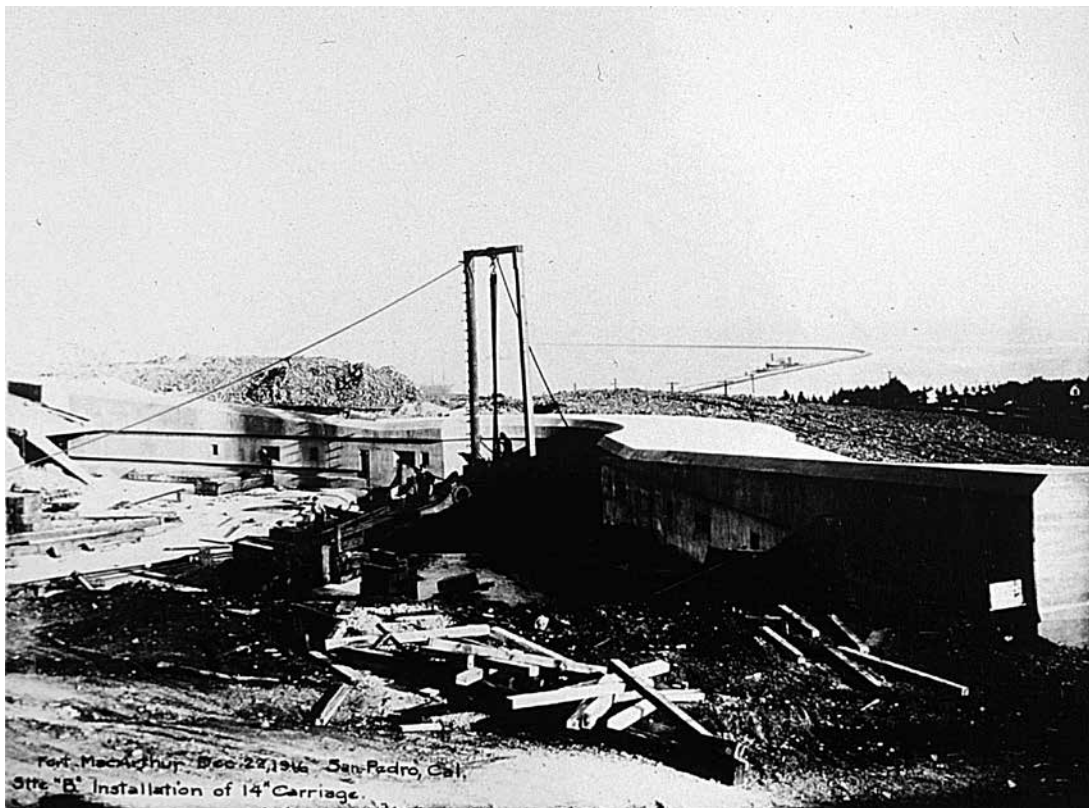
Construction of a 14-inch gun battery at Fort MacArthur, 1916 (US Army Corps of Engineers photo)
