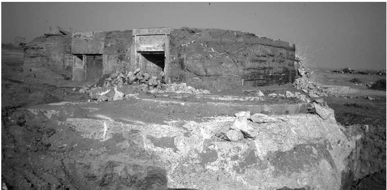
Battery Harrison (BCN 242), Bolsa Chica, being demolished 1993 (photo by Mark Berhow)
