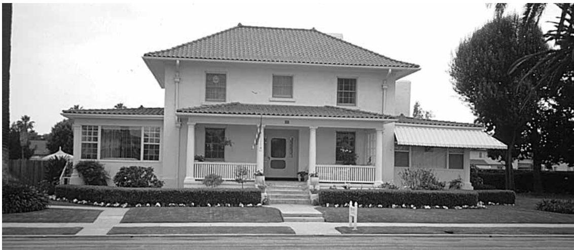
Officers Quarters, Middle Reservation, Fort MacArthur 1996 (photo by Mark Berhow)
