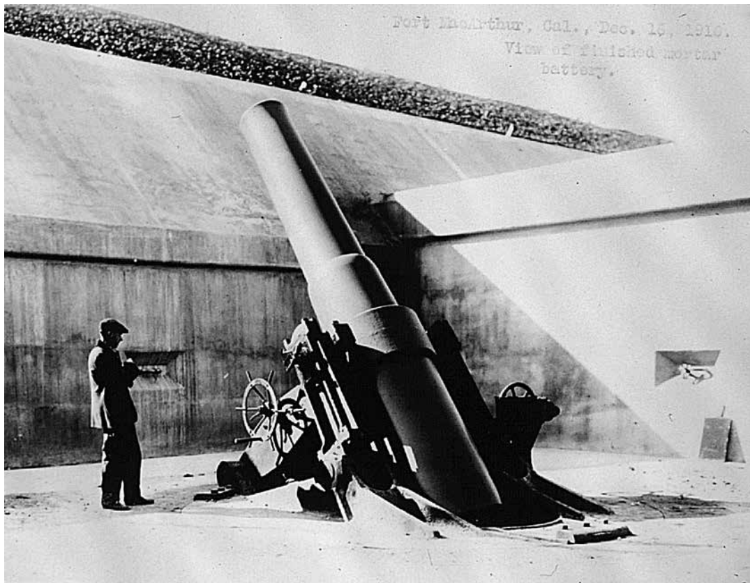
Battery Barlow-Saxton, 1916 (US Army Corps of Engineers)
