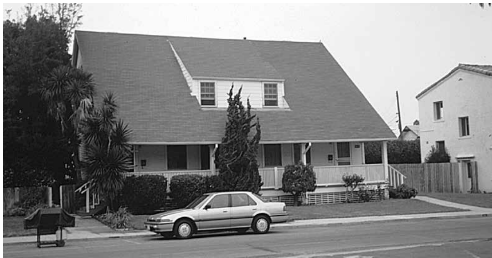
Non-Commissioned Officer's Quarters (duplex), Middle Reservation, Fort MacArthur 1996 (photo by Mark Berhow)
