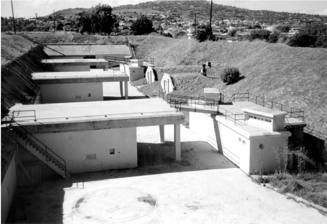
Battery Barlow-Saxton 1999 (photo by Mark Berhow)
