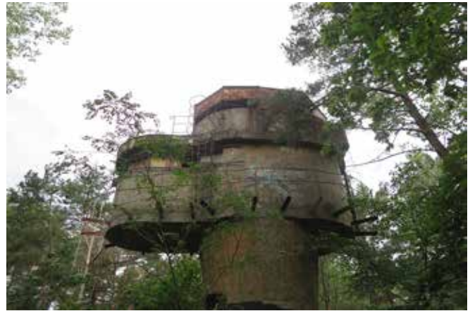
The rangefinder and periscope viewfinder positions of the 27th Fixed Artillery Battery's Fire Control Tower
