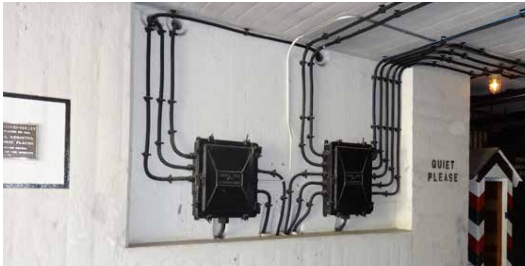
Fuse boxes for the electrical system at Battery Osgood-Farley, 2016 (Mark Berhow)
