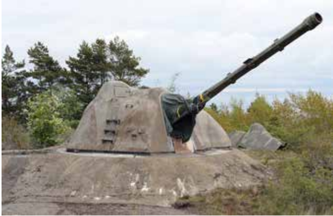
Landsort Battery 12cm/m70 turret (CHB) and magazine
