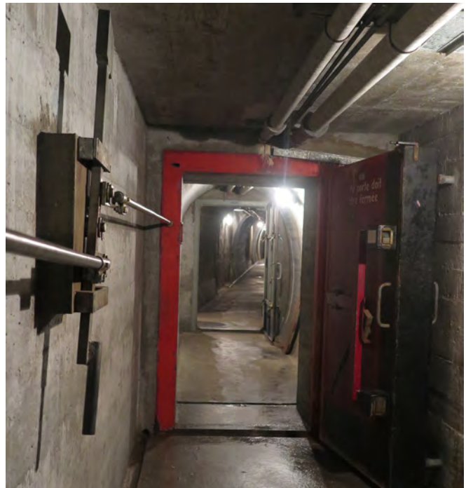
Protective door system between barrack area and gun casemates at Fort Champex C. Penfold
