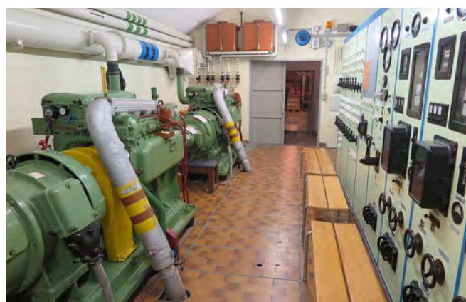
Power room with Sulzer motor generators and switchboard at Festung Naters C. Penfold
