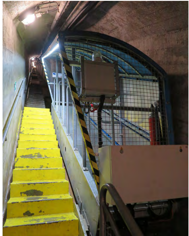
Cableway transport inside Festung Sasso da Pigna that moved personnel from the accommodation level to the artillery casemate, more than 400 steps. C. Penfold
