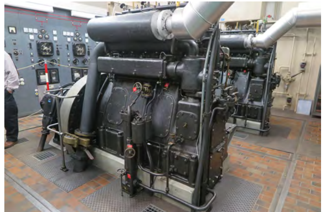
Three ready-to-go Sulzer motor generators in the power room at Festung Furggels. C. Penfold
