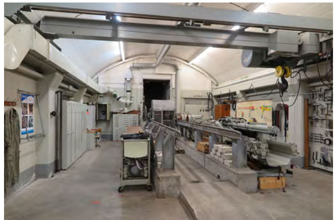
Turret support chamber with crew lift and spare barrel with access shaft to turret at Battery T1 C. Penfold
