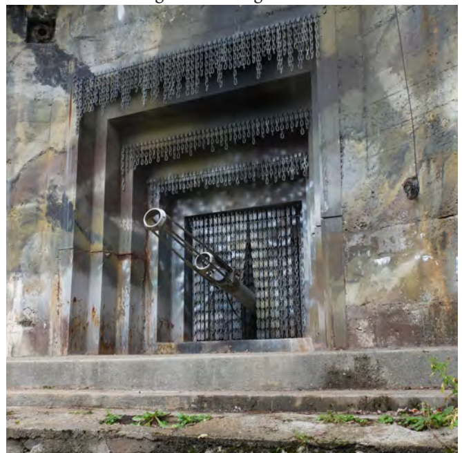
The exterior of the 10.5 cm casemate with the barrel fitted with a velocity gauge at Festung Crestawald. T. McGovern.
