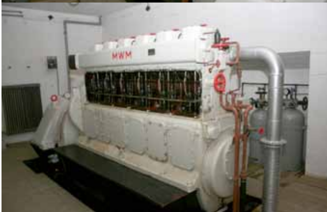
Two of several motor generators to power the gun emplacement
