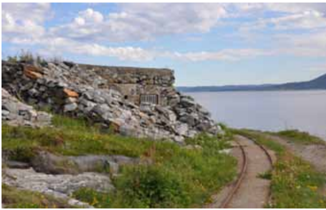
Hambaara Fort – 60 cm rail line to move 53cm torpedoes to the launcher on the edge of fjord
