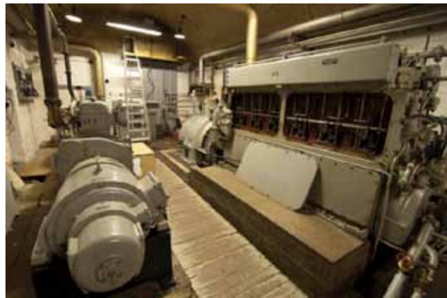
Austrått Fort – Power room for the 28 cm SKC/34 triple turret – diesel motor generator
