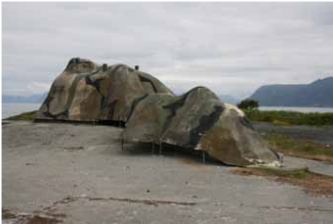
12cm L/70 gun at Meløyvær Fort - Fiberglass camouflage in place
