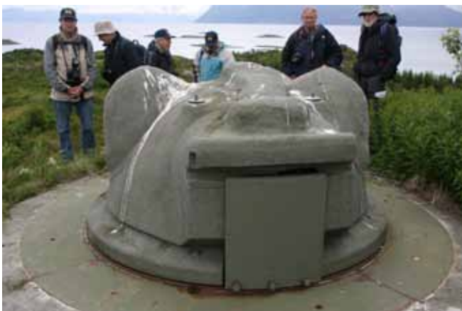
Armored turret for the 12/70 laser rangefinder – another photograph stand-off!
