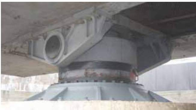
Central Pintle in Emplacement #2 at Battery Vara, Movik Fort
