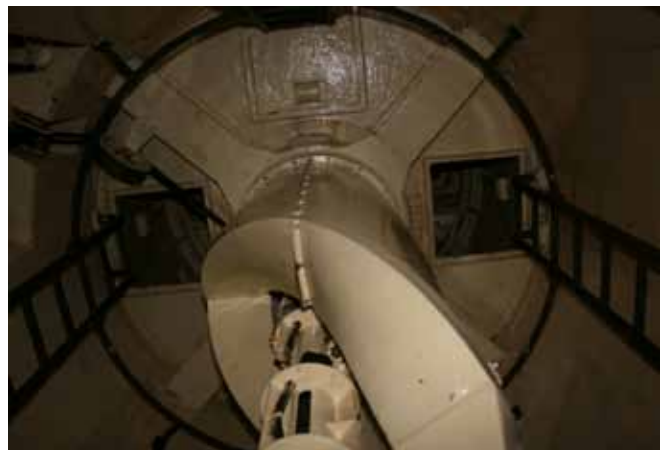
Elevator/Shaft for Fixed Ammo to reach 75mm Turret – Eastern Position – Bolaerne Fort – June 11, 2013
