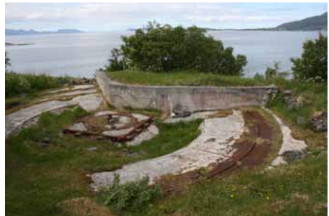
German “Panama mount” emplacement at HKB 13./983 Elgsnes for one 15.5 cm K418 (f) gun
