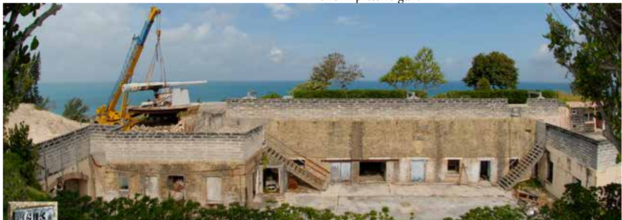
Fort Victoria and 9.2-in gun with the barrel lifted clear of the mounting (EH)
