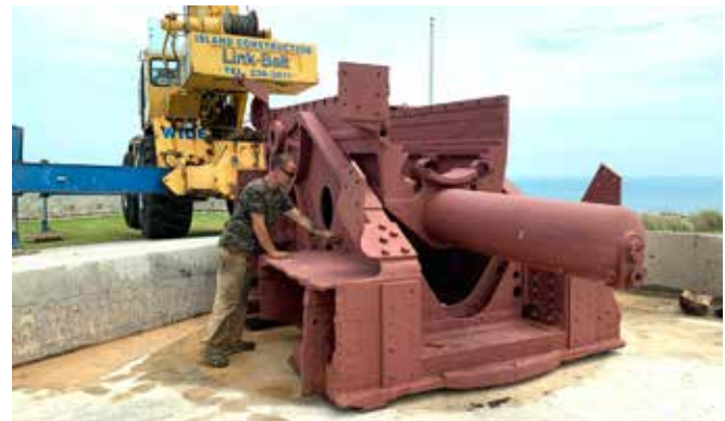
Cradle and carriage are re-joined, in position. 22.04.21 (MT)
