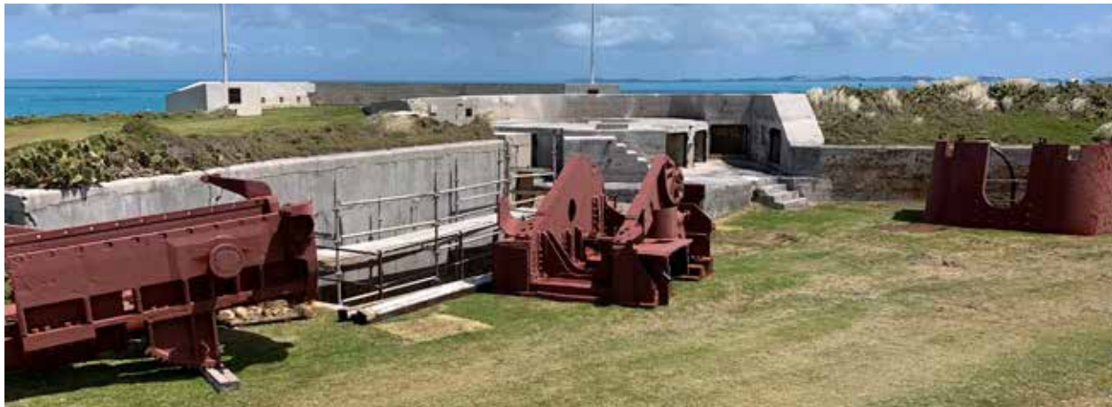
Gun components with red undercoat ready to be installed. 8.04.2021 (NMB)
