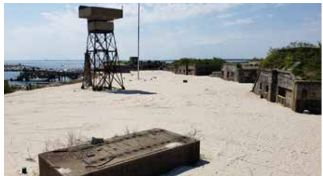
The cleared Parade Ground with the WW2 BC Tower. Note how the CRF station on top is leaning down due to the failure of the steel supports in the observation windows.
