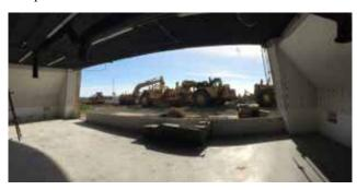
Navy contractors have removed the earthen cover on Battery 134 and started concrete demolition in April (see photos below). Per the agreement with the State Historic Office and CDSG, the navy is documenting the Fort Emory buildings and will include demolition pictures in the final documentation report.
