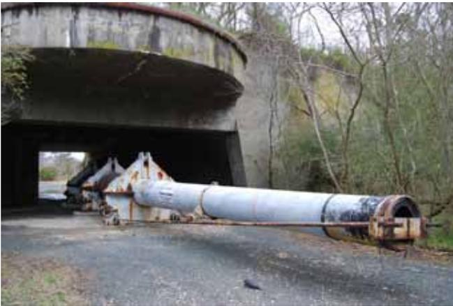
The 16-inch barrel in place in Battery Winslow. The top of the cradles will be removed.
