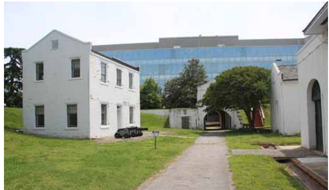
The entry gate with headquarters building/ commanding officer's quarters on the left and navy arms storage building on right. Beyond the arms storage building is an auxiliary building.
