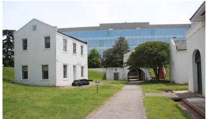
The entry gate with headquarters building/ commanding officer's quarters on the left and navy arms storage building on right. Beyond the arms storage building is an auxiliary building.
