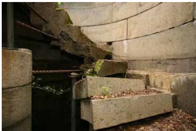
North staircase before
