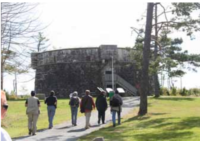
Prince of Wales Tower
