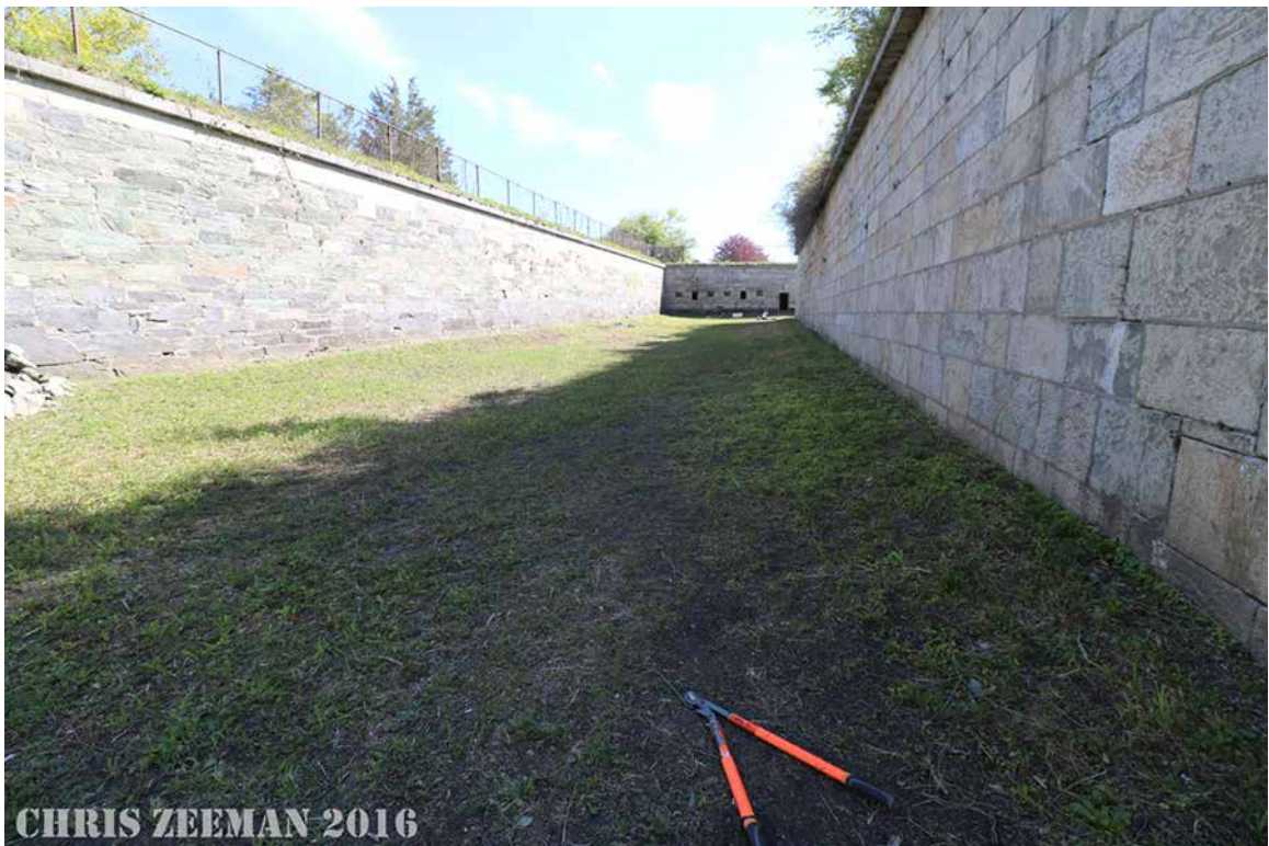
Fort Adams Redoubt Ditch
