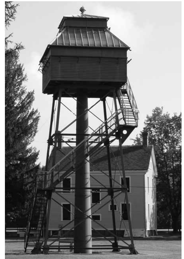
Fire Control Tower and Administration Building Fort Mott State Park, New Jersey
